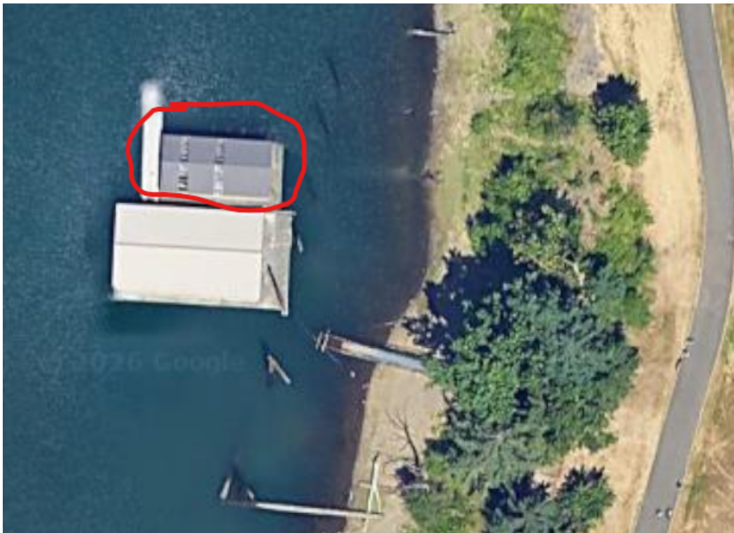
Photo 20 – Structure that was Removed
