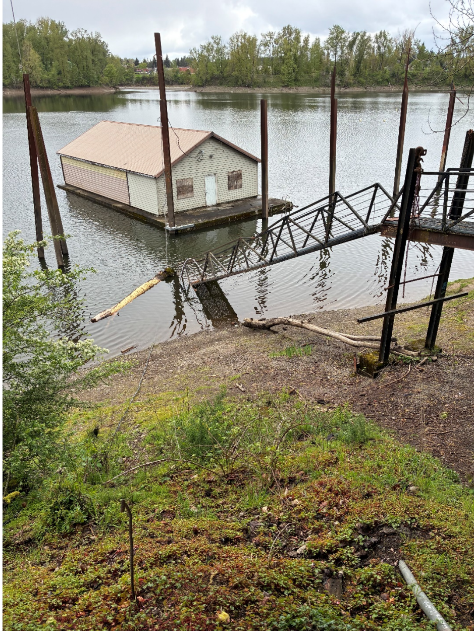
Photo 20 – Structure that Remains
