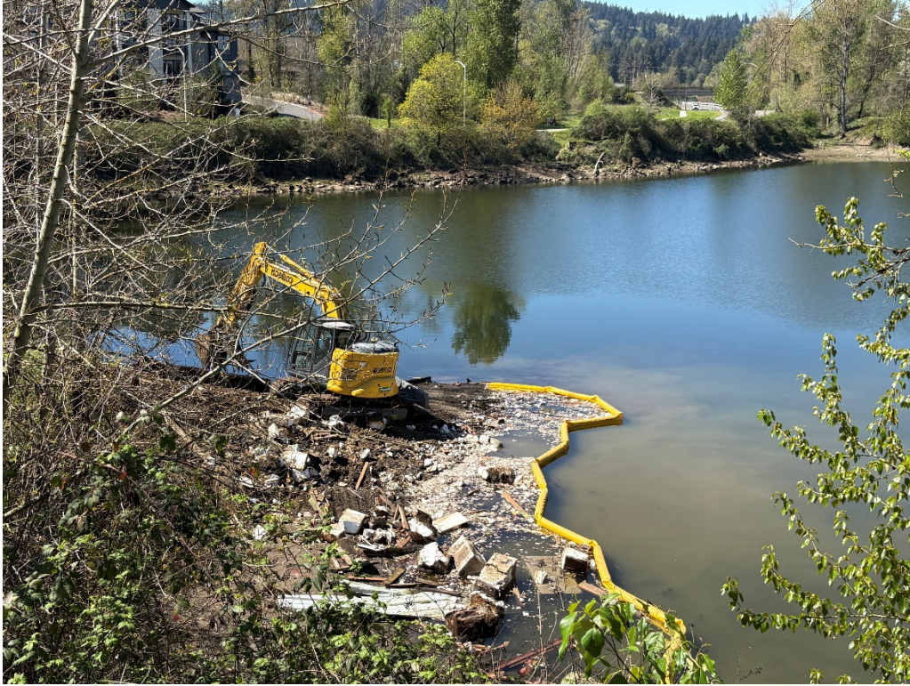
Photo 4 – April 8, 2026 – Cleaning up Water after Removal
