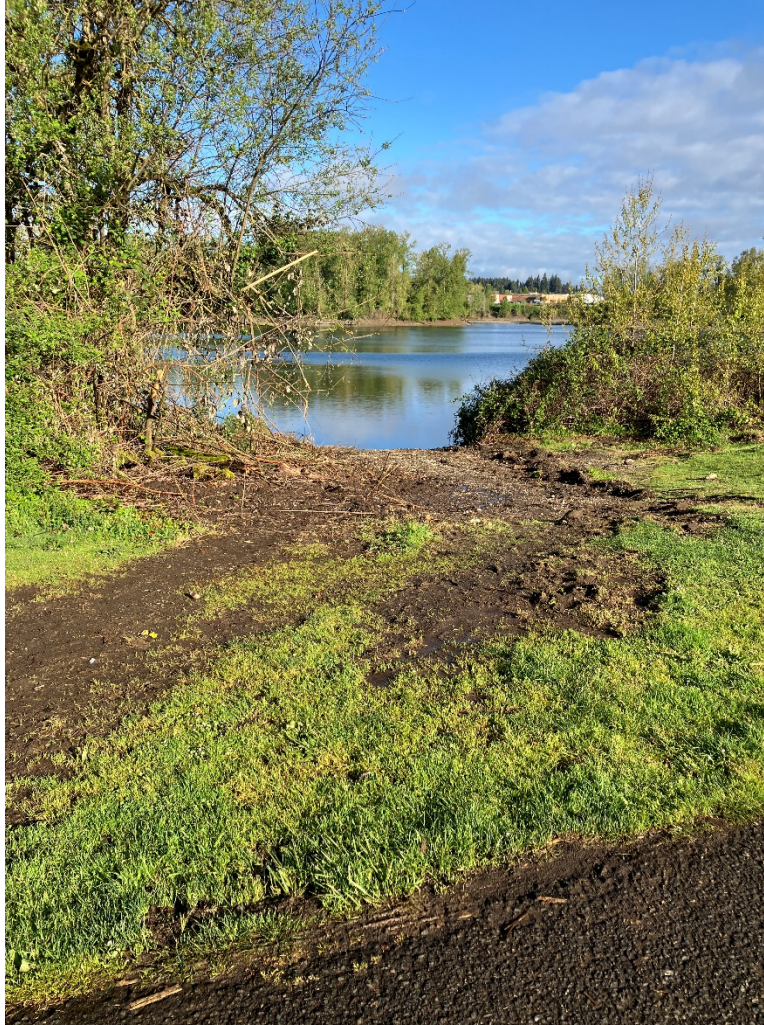
Photo 11 – April 16, 2026 – Removal Path & Damage
