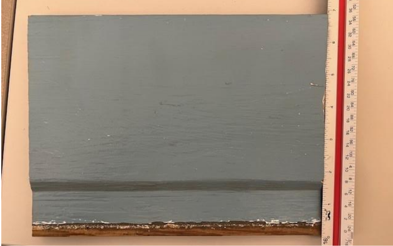
Existing wood siding sample showing 6.5-inch reveal and 1-inch channel
