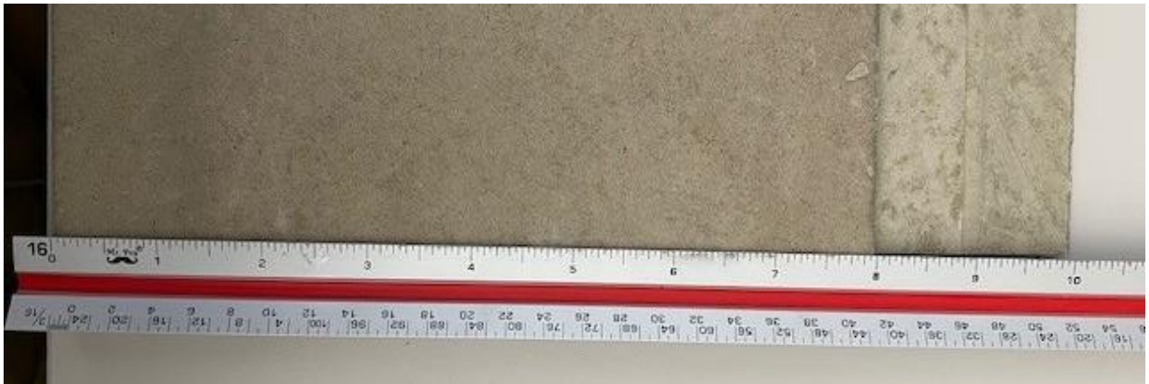
Sample B Plan View showing 9-inch reveal and 1-inch channel on the right
