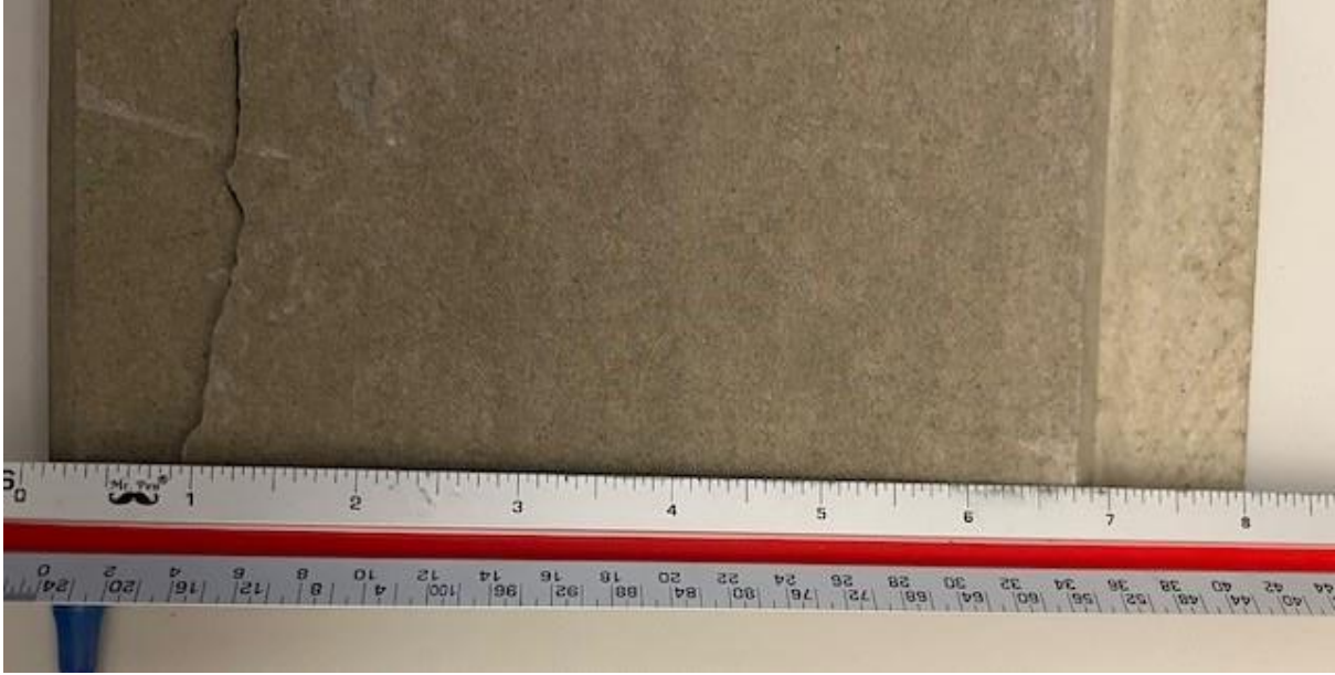
Sample A Plan View showing 8-inch reveal and V-groove on the left
