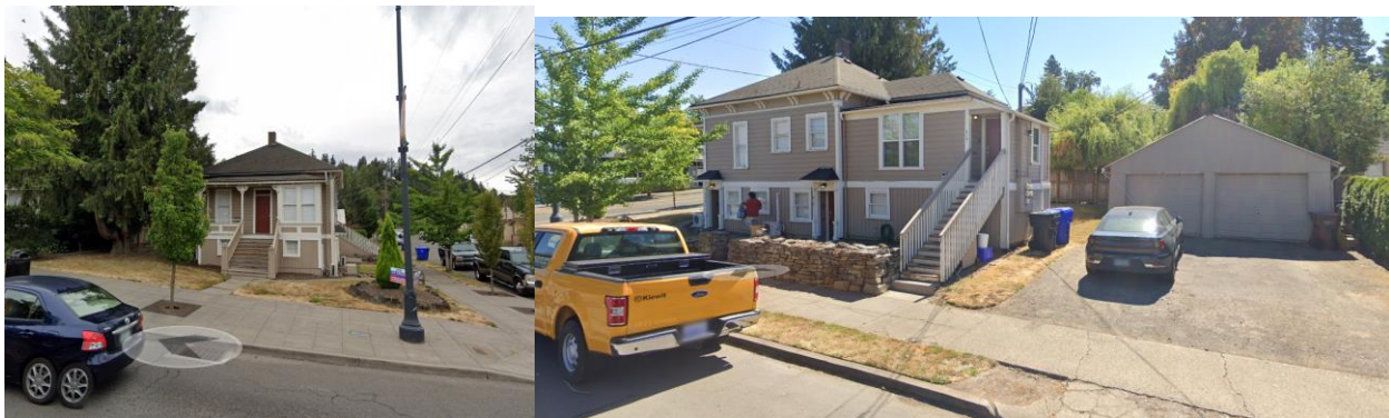
Street Views looking SW from 7 th Street (L) and SE from JQ Adams Street (R), courtesy Google Maps
