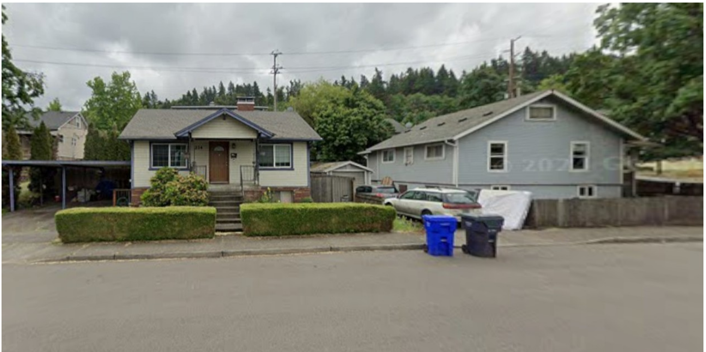
FIGURE 3. STREET VIEW (2024) 313 S 2nd St (side elevation) and 314 Tumwater
