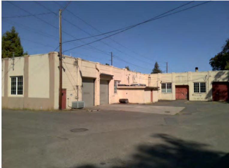
Back view of building from within the site
