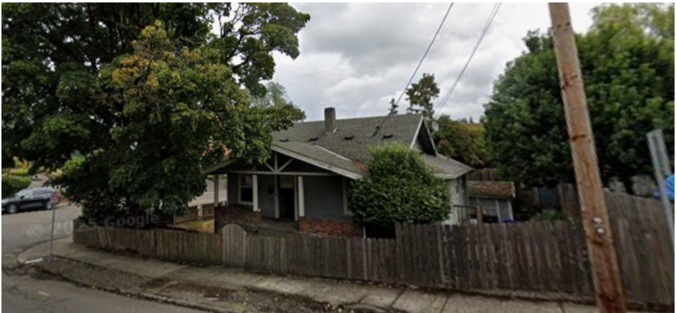
FIGURE 4. STREET VIEW (2024) 313 S 2nd St
