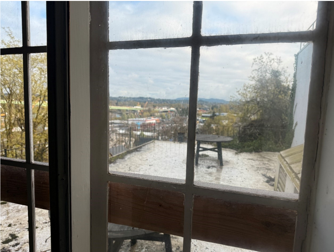
Figure 8 Looking northwest at the location of the window removal and door replacement at the lower deck. Note historic metal window .
