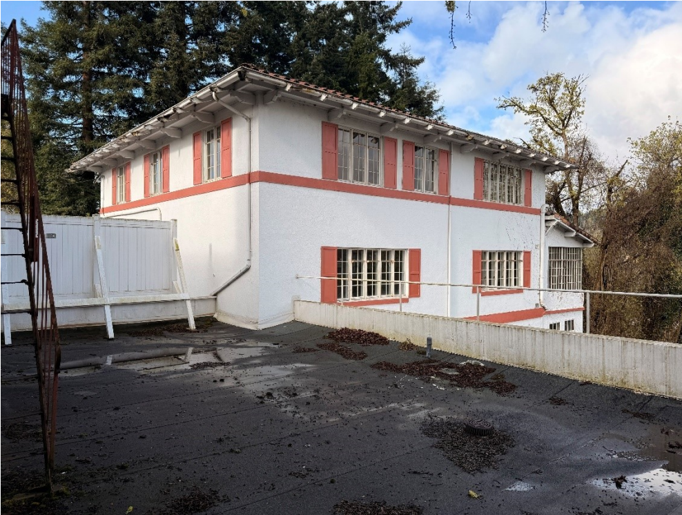
Figure 7-Looking southwest at the location of the proposed connector hallway (fence location on upper deck)
