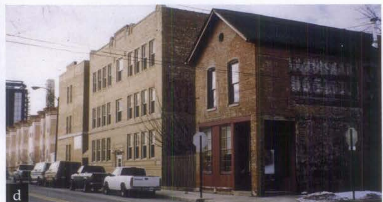
Figure 5. This addition (a) is constructed of matching brick and attached by a recessed connector (b) to the 1914 apartment building (c). The design is compatible and the addition is smaller and subordinate to the historic building (d).
