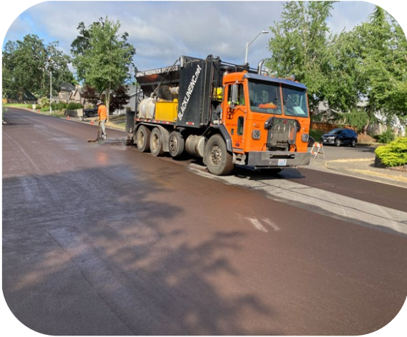
Slurry Seal Treatment
