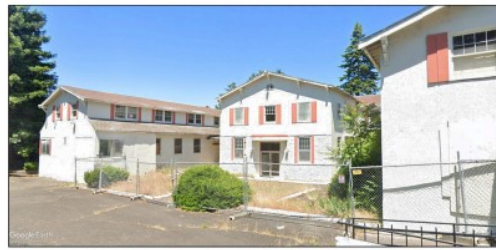
3 EXISTING VIEW AT 10th ST. DATE: 2006
