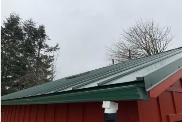
7 RESTROOM ROOFING, METAL
