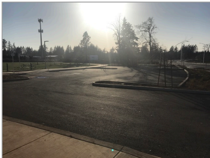
Overview of accessible parking area
