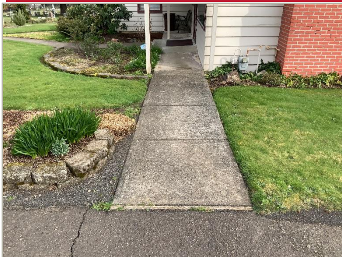
1 – EXTERIOR PATH OF TRAVEL TO BUILDING ENTRANCE
