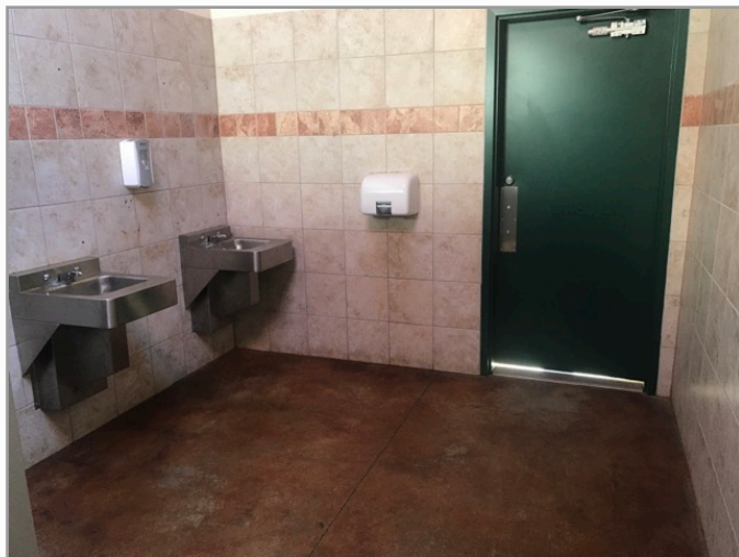
Toilet stall overview
