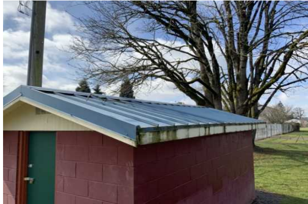
8 PUMP HOUSE ROOFING, METAL
