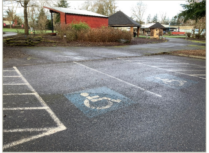
2 - MISSING PARKING SIGNAGE
