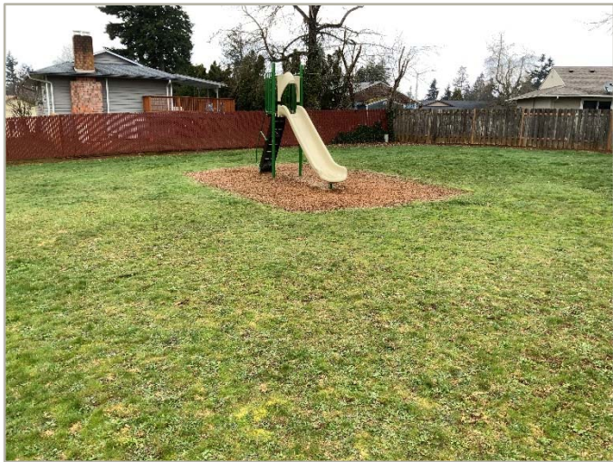
3 – NO ACCESSIBLE PATH TO PLAY STRUCTURE
