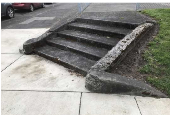
47 DETERIORATED STAIRS
