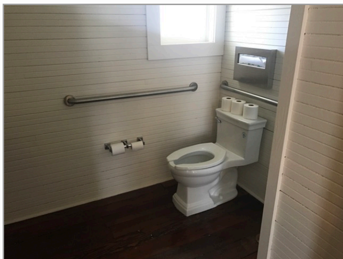
Toilet stall overview
