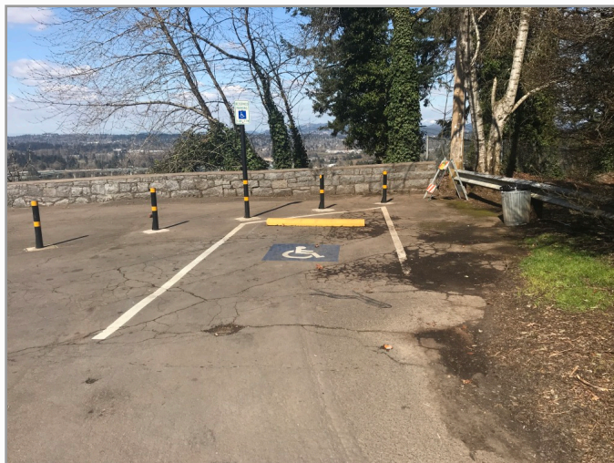
Overview of accessible parking area
