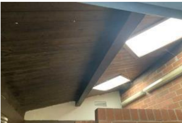
11 CEILING FINISHES, WOOD PANELING
