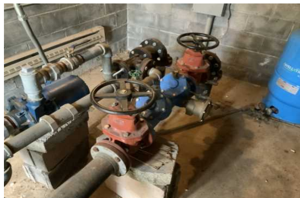
16 BACKFLOW PREVENTER, DOMESTIC WATER
