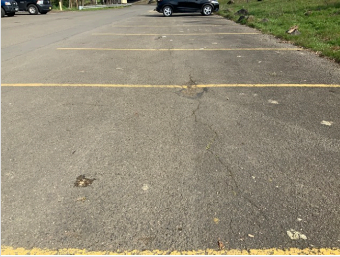
Overview of accessible parking area
