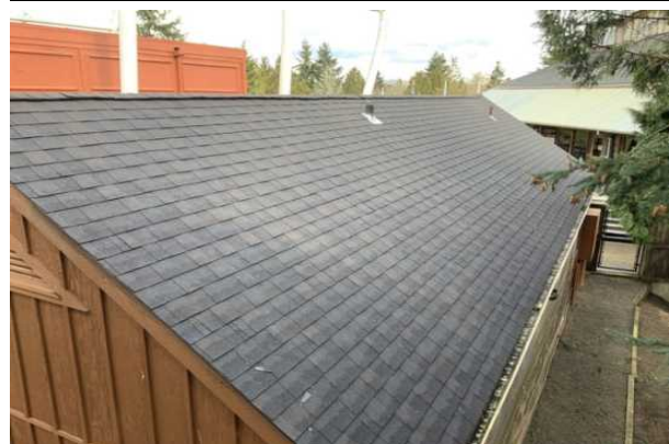
12 ASPHALT SHINGLE ROOF
