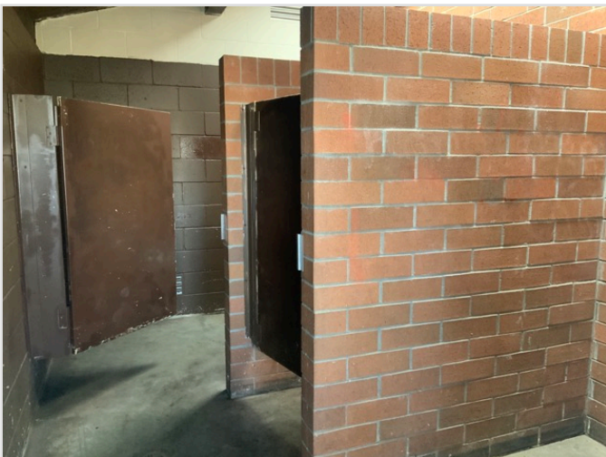
Toilet stall overview
