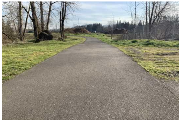
9 TRAIL SURFACE, ASPHALT
