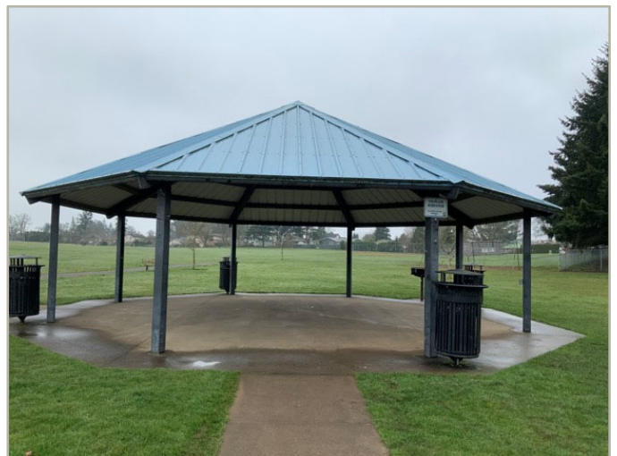
12 – ACCESSIBLE ROUTE TO PICNIC SHELTER
