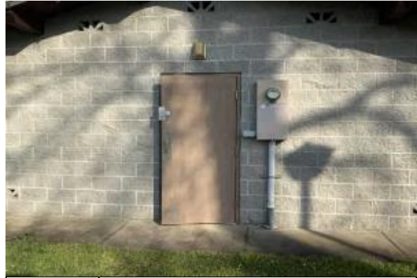
8 EXTERIOR DOOR, STEEL
