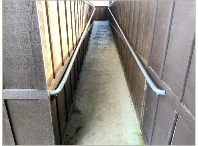
2 – RAMP TO BUILDING ENTRANCE
