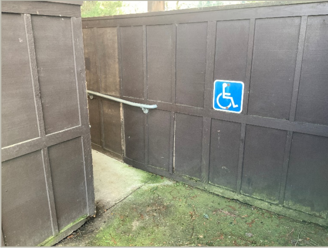
1 – EXTERIOR ACCESSIBLE PATH
