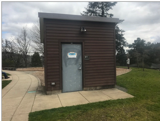
Toilet stall overview
