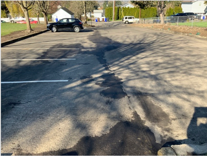
Overview of accessible parking area
