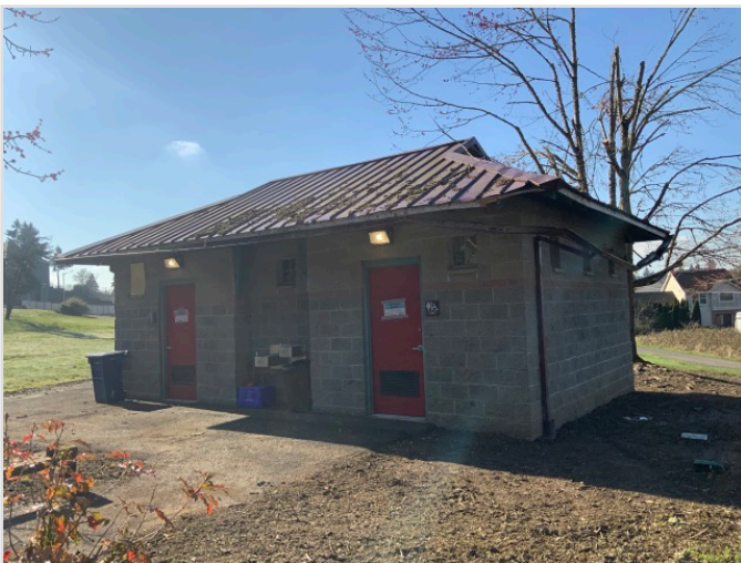
Toilet stall overview
