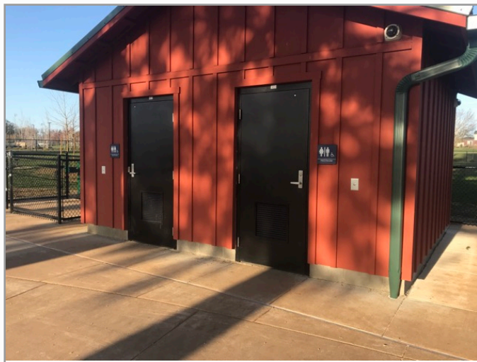
Toilet stall overview
