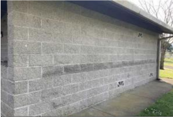
7 EXTERIOR WALLS, CONCRETE BLOCK
