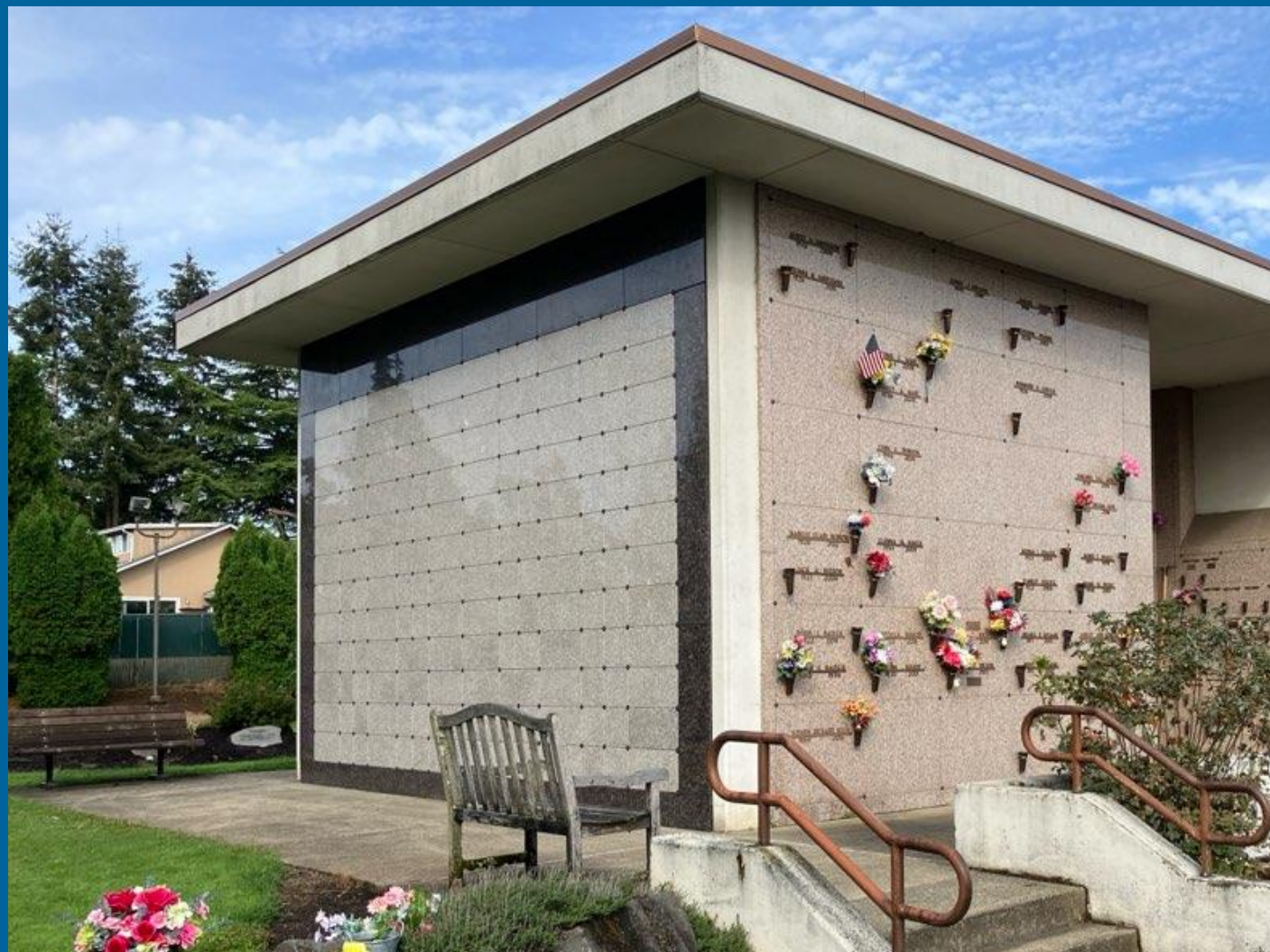
New Niche Wall Columbarium install in 2024
