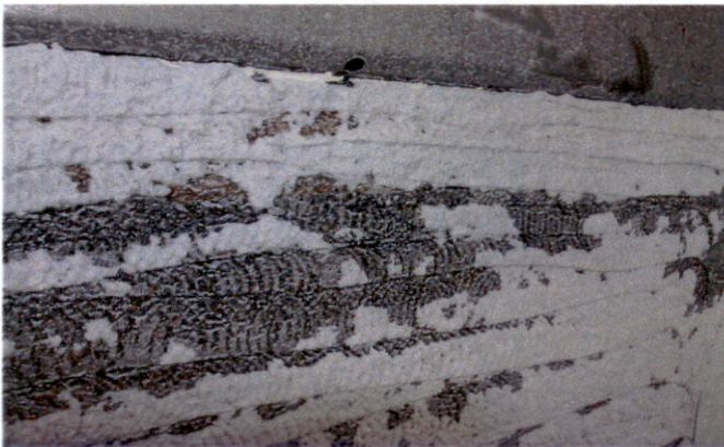
Pool Surface After Hydro-Blasting
