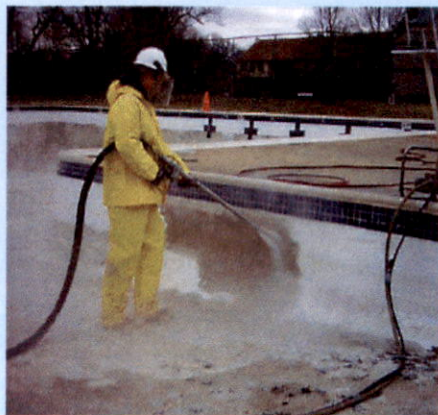
Hydro-Blasting in Action
