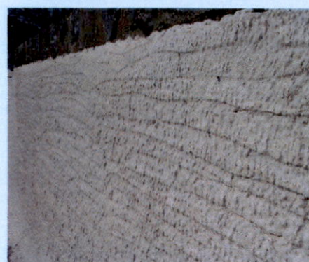
Residential Plaster Prep Overland Park, KS
