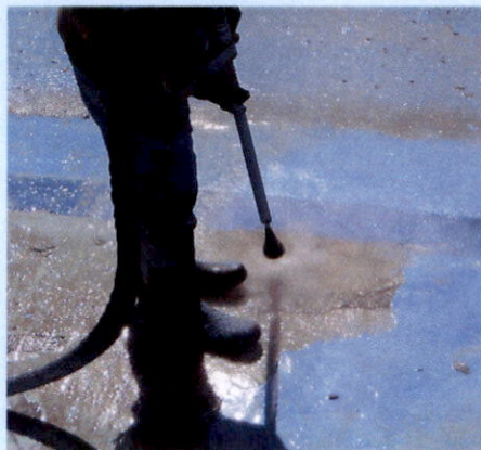
Hydro-Blasting in Action
