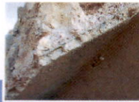
Plaster aqueduct interior
