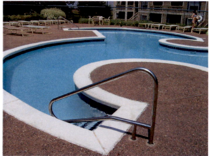
Pool re-plastered by Mid-America Pool Renovation, Inc.
