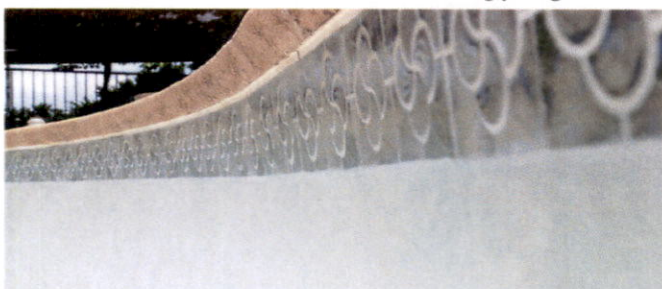
New plaster flush with tile. No ugly bulge.
