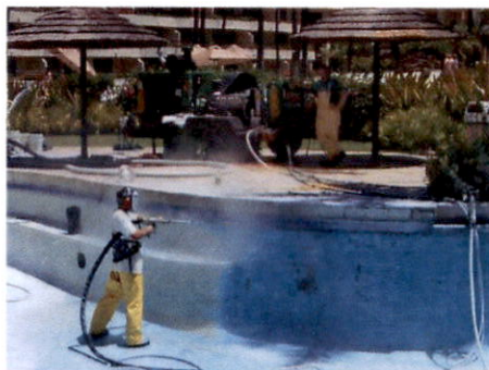
Hydro-Blasting removing pool paint
