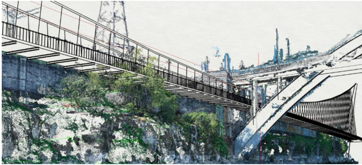
Figure 10. The Fully External Alignment Threading Through the Historic Arch Bridge
