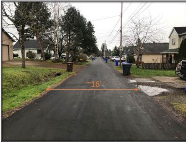
Figure 2-5: Narrow Roadway (Hiram Ave)
