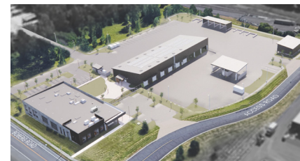
Wilsonville Public Works
