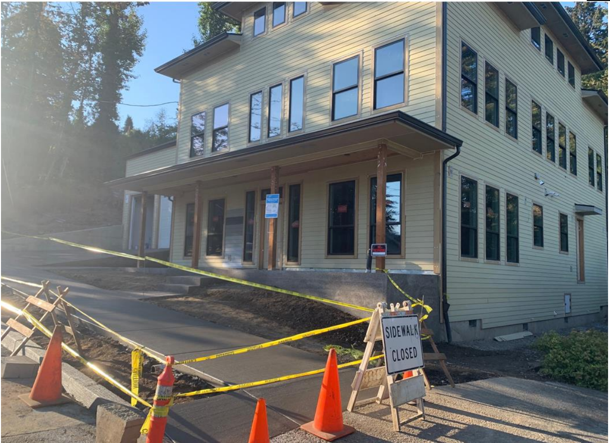
Figure 4 Existing condition of front and side elevations.- September 20, 2022
