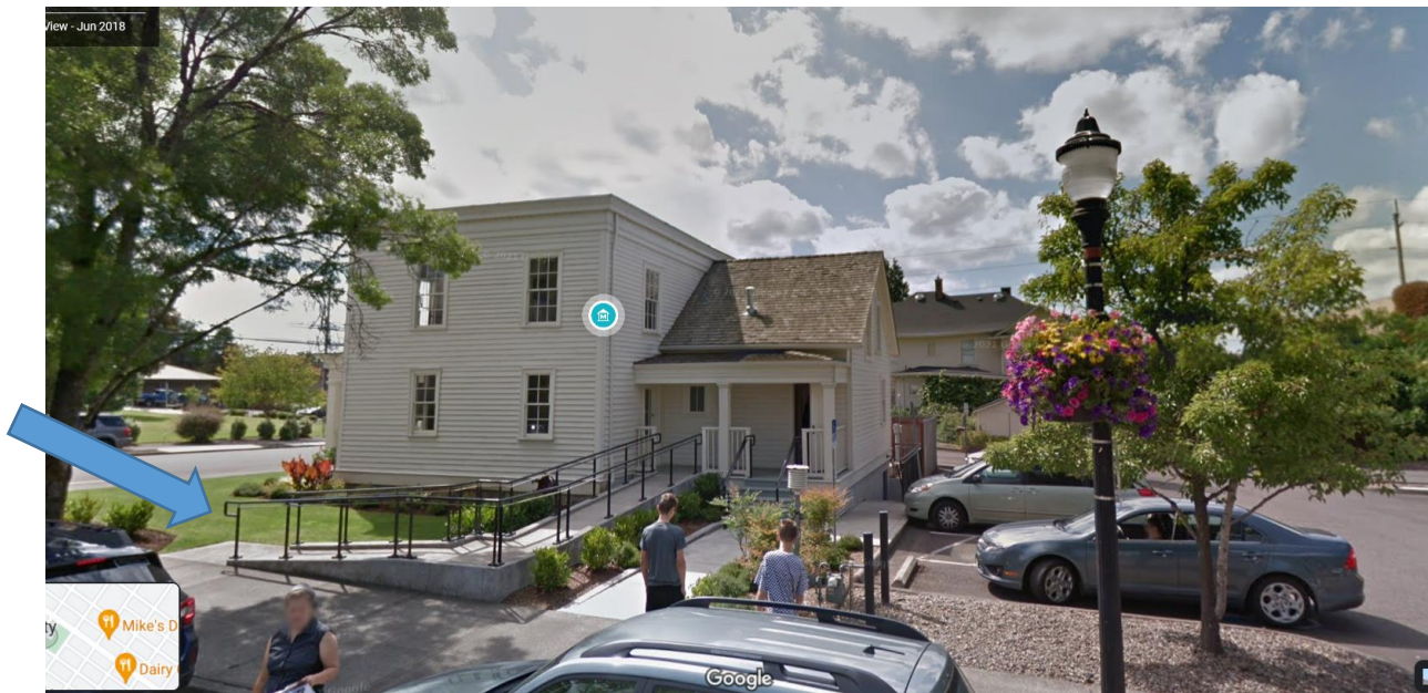
619 6 th Street Ermatinger House ADA ramp (2014)
