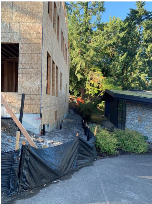
Figure 4 Existing condition of exposed foundation- September 21, 2021
