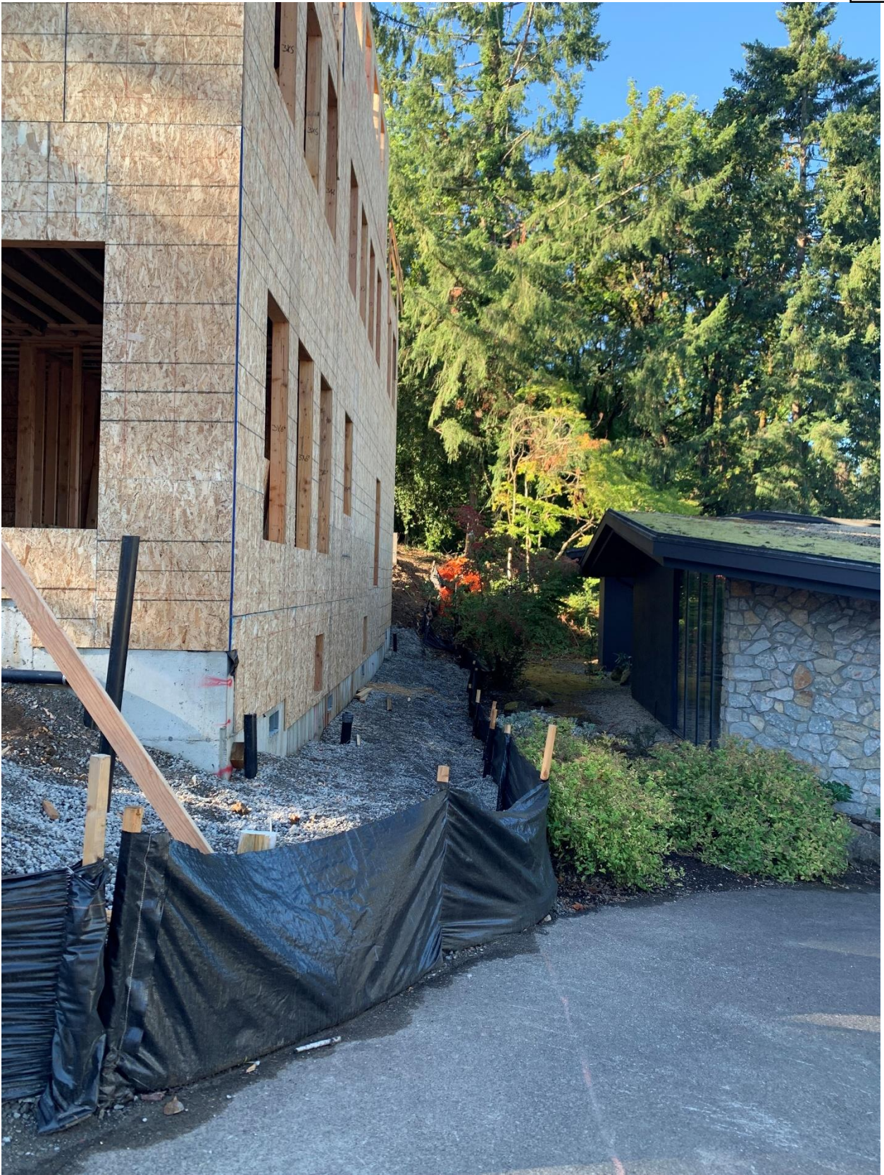
Figure 4 Existing condition of exposed foundation- September 21, 2021
