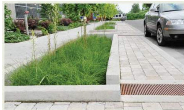
Beaumont Village Lofts, NE Portland
