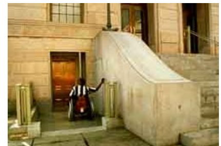
A new elevator entrance was provided next to the stairs to provide universal access to the services inside. Photo: Courtesy, GSA.
