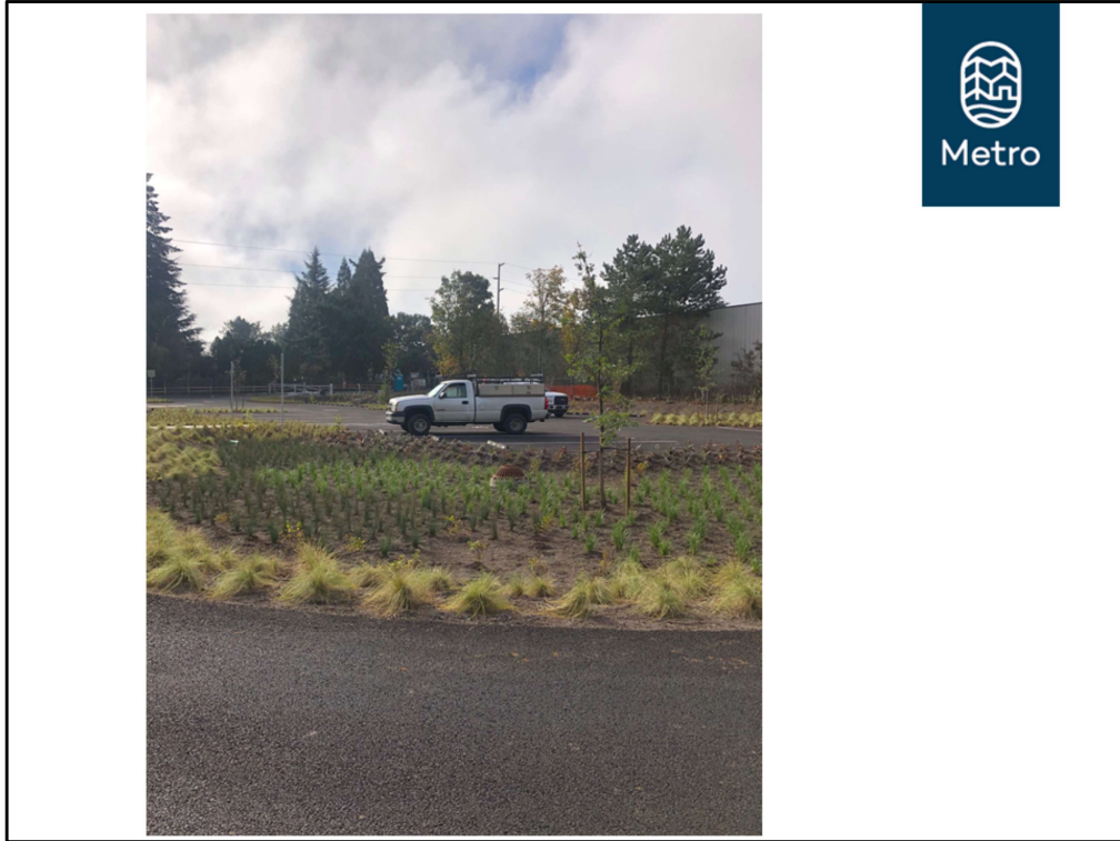
A view of the parking facilities and storm water management swales.
