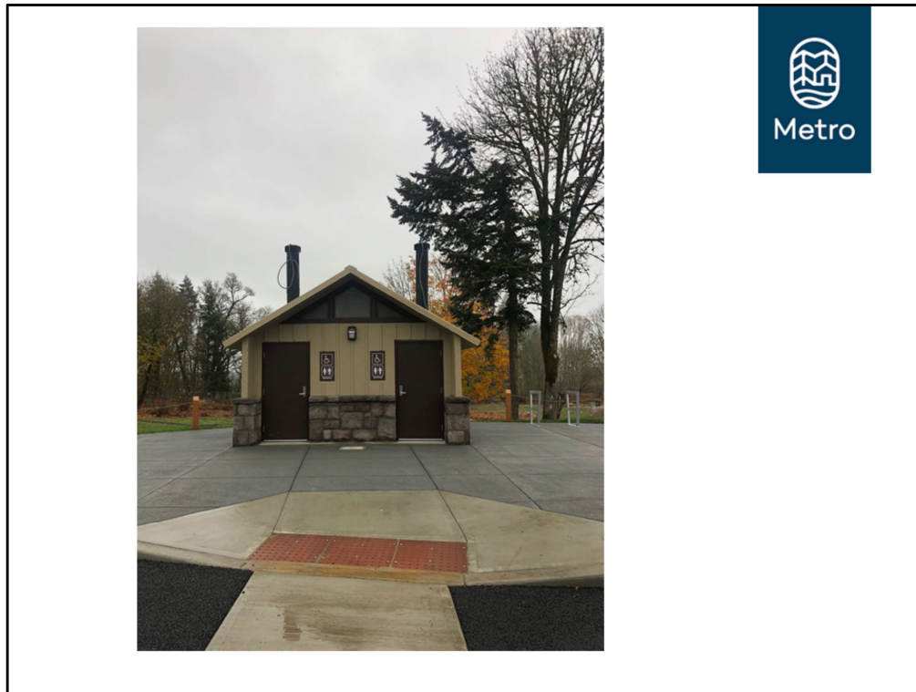
A look at the recently installed double stall, vault bathrooms.
