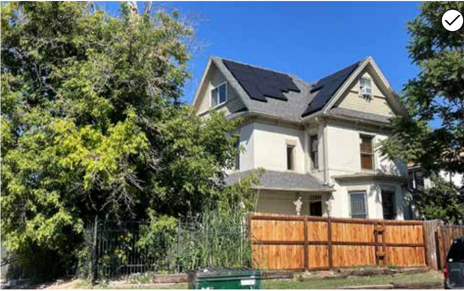
40. Solar panels are placed to avoid obscuring distinctive roof features.
