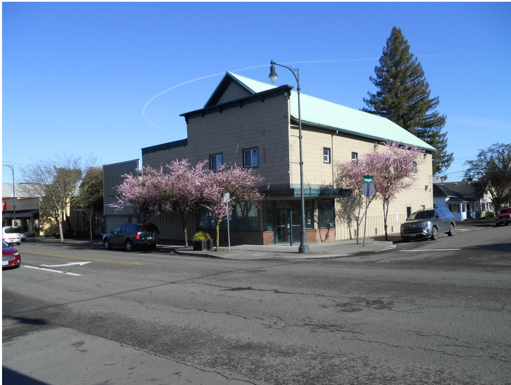
Front Building Corner
