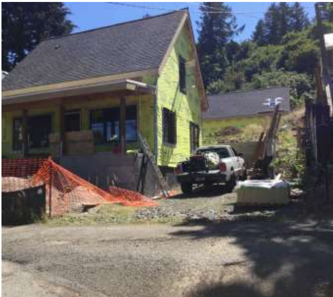
(Left) View from right-of- way on 4 th Avenue – House #2 skylight. August 2020
