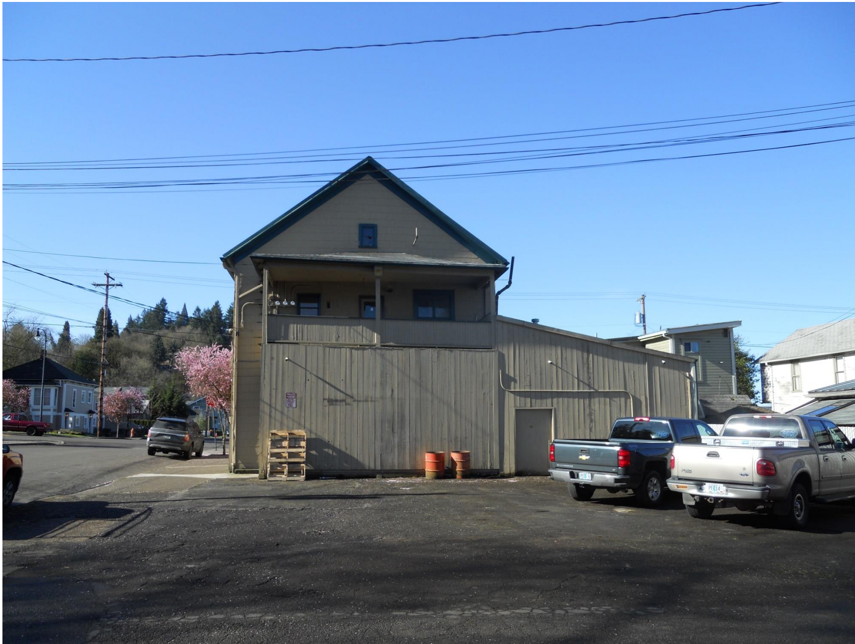
Back of Building
