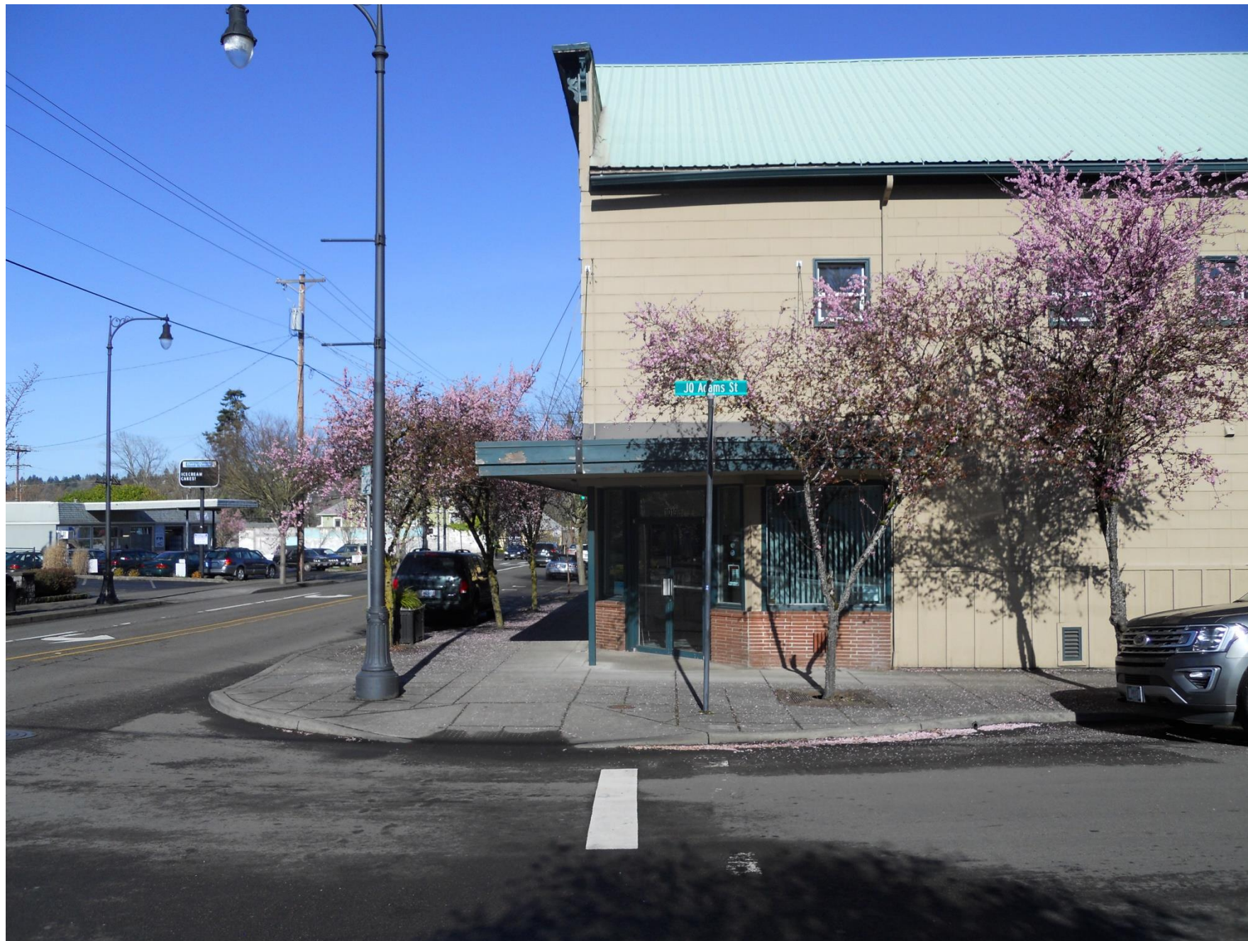
Front Corner of Building
