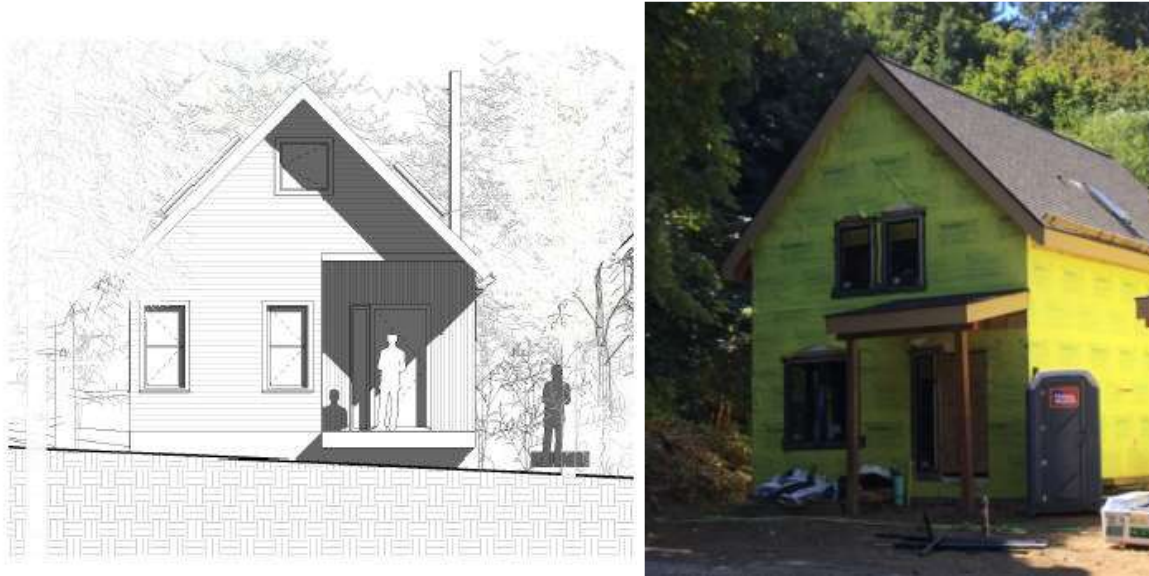
Proposed and constructed versions of House #5. The height difference is approximately 4.5 feet.
