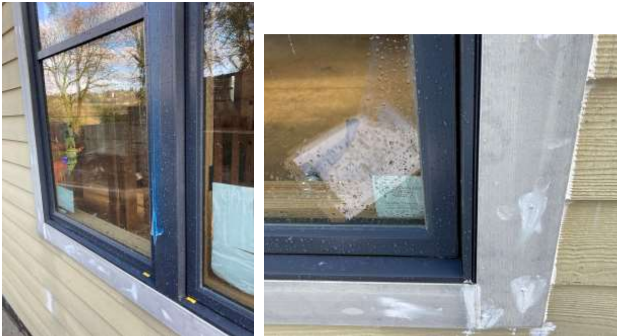
Casement windows with simulated divided lite on the front of House #1.
