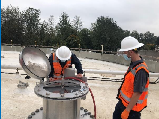
Inspecting the new Digester: Operators look through the new digester view port to verify mixing.
