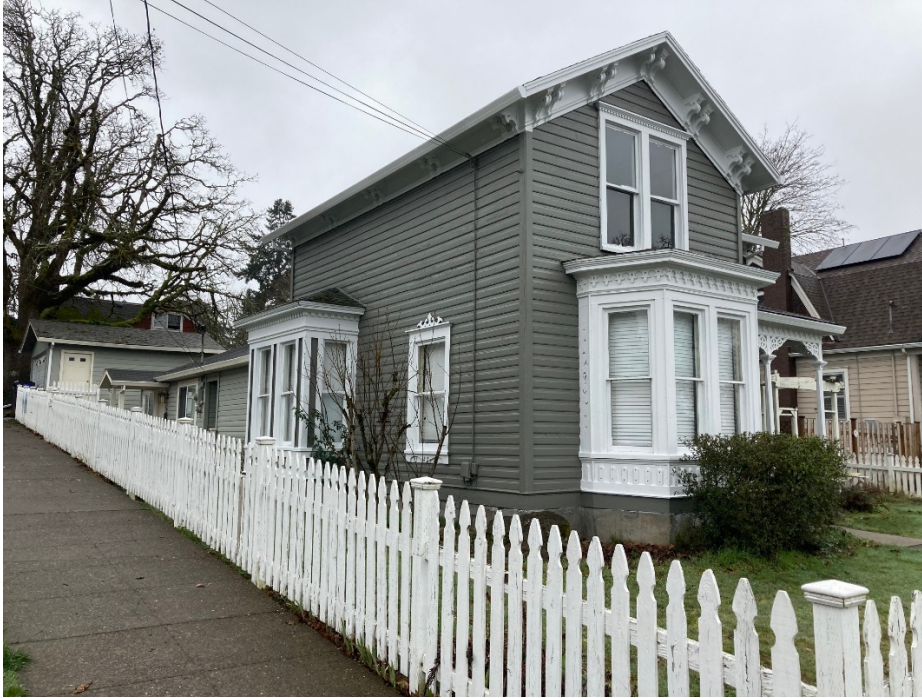
Figure 3: Existing Conditions – Frederick White House from Corner of 10 th and Jefferson
