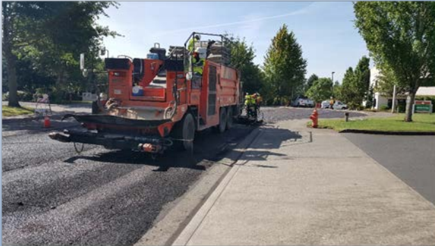
Micro Seal Application along Beavercreek Road
