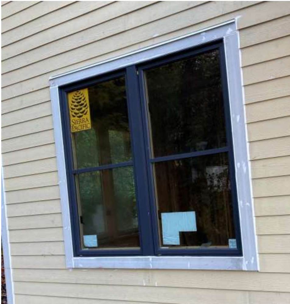
Casement windows with simulated divided lite on the front of House #5.
