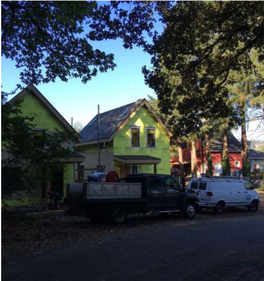
View from right-of- way on Miller Street – House #4 skylights are visible. August 2020
