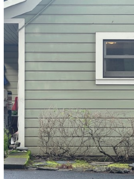
502 4th Ave Siding
