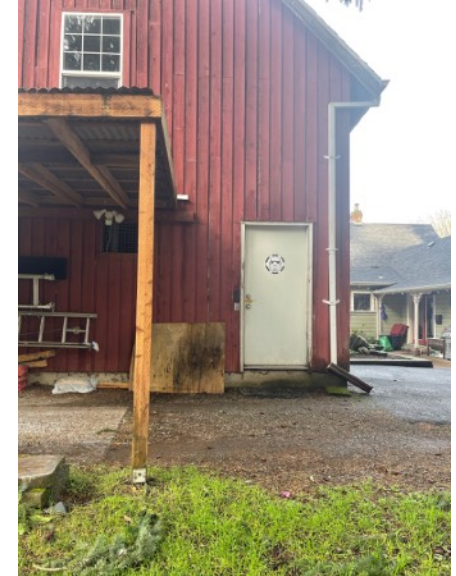
502 4th Ave Siding
