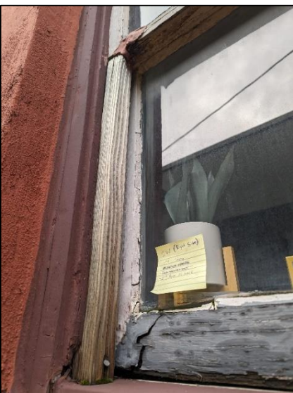
Figures 7 through 13- Details of existing windows condition and visible deterioration.
