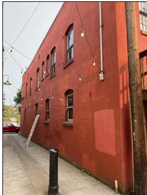
Figure 3- Alley view of southwest (right) elevation
