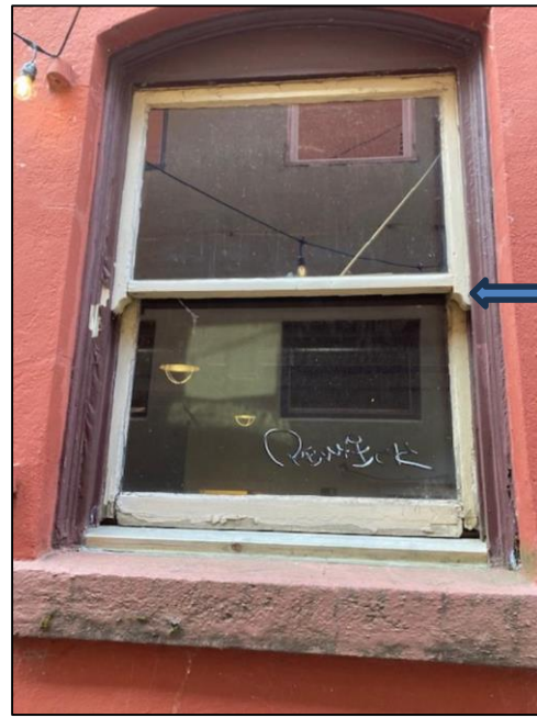
Figure 5 – Typical Double-Hung Window
