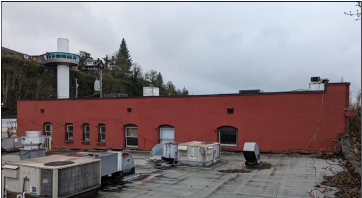
Figure 6- Adjacent property view of northeast (left) elevation
