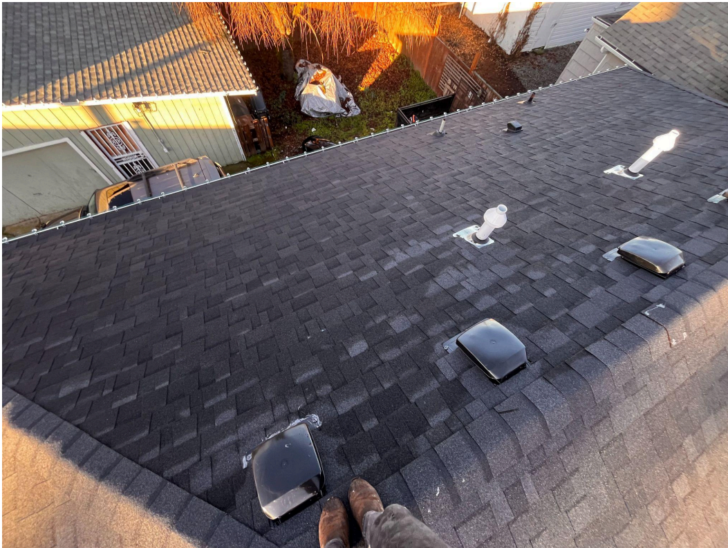
Back Roof Section
