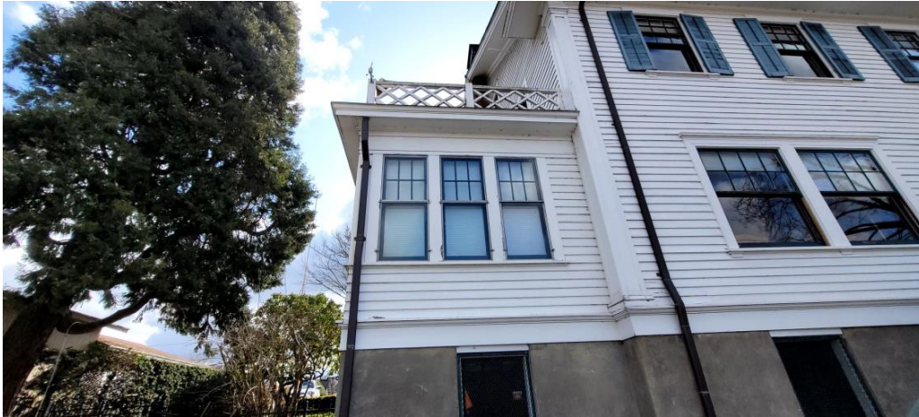
Northwest corner of home with sun porch roof
