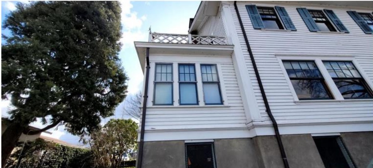
Figure 4-northwest corner of the home with sun porch
