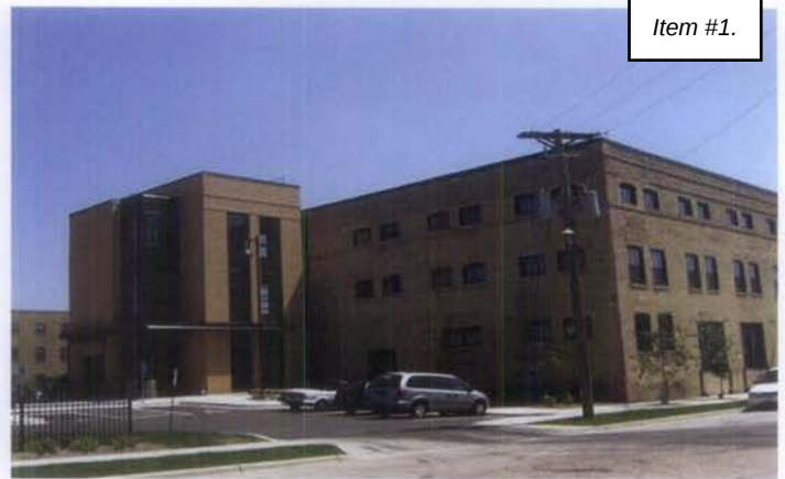
Figure 8. The rehabilitation of this large, early-20th century warehouse (left) into affordable artists' lofts included the addition of a compatible glass and brick elevator/stair tower at the back (right).
