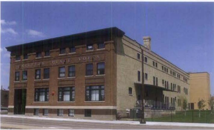
Figure 8. The rehabilitation of this large, early-20th century warehouse (left) into affordable artists' lofts included the addition of a compatible glass and brick elevator/stair tower at the back (right).
