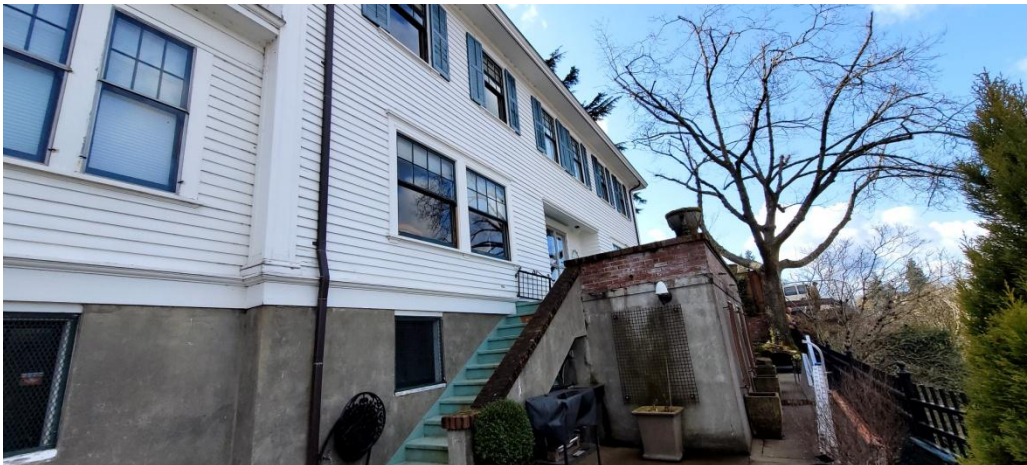
Northwest corner of existing main level porch/ basement
