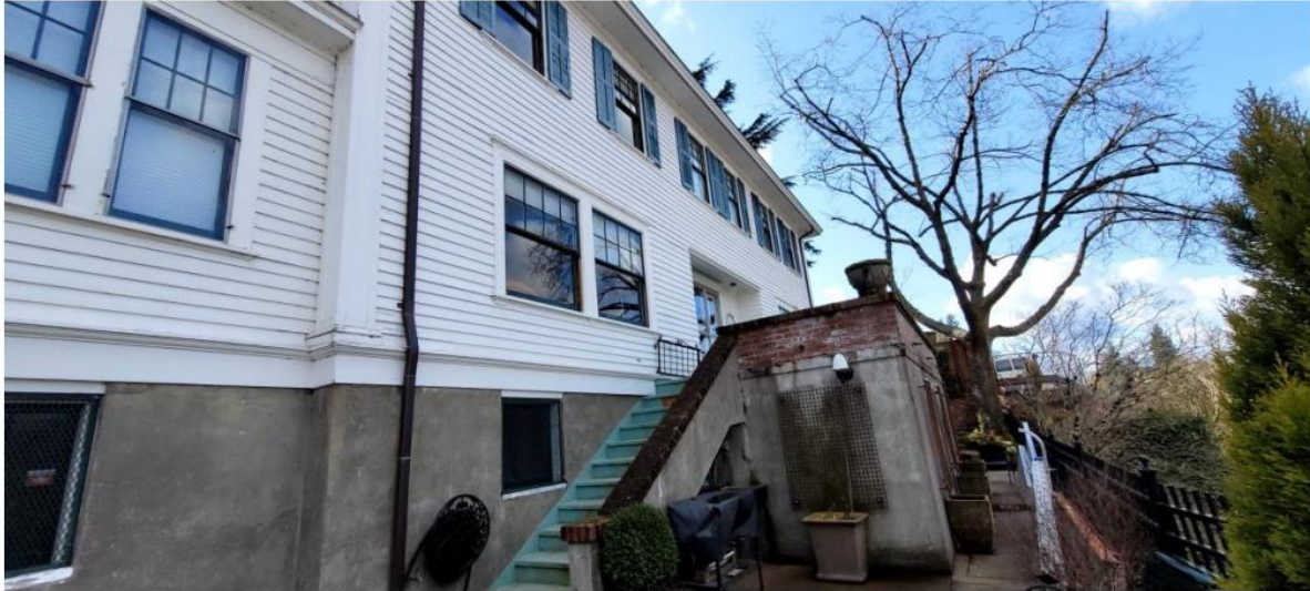
Figure 3- Northwest corner of existing main level porch/basement
