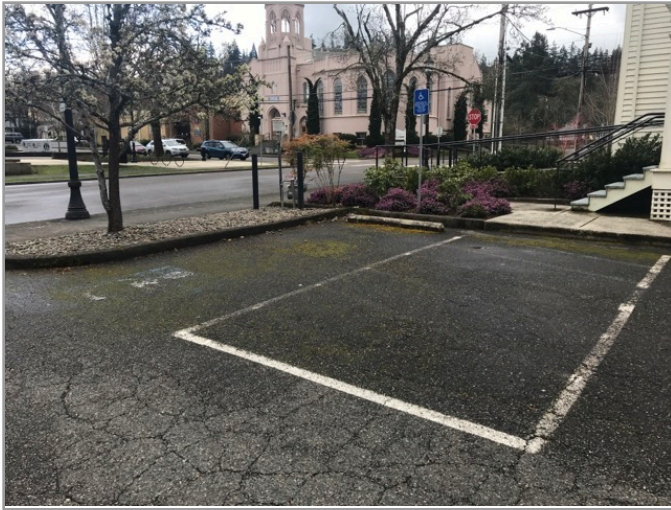
Overview of accessible parking area
