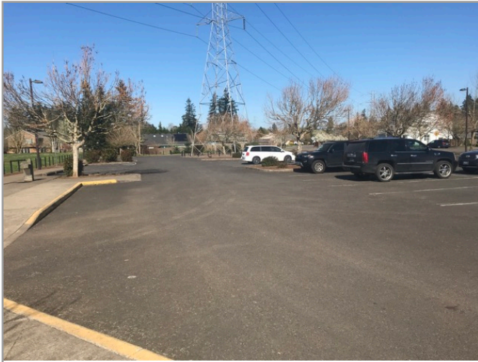
Overview of accessible parking area
