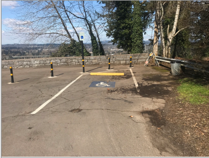
Overview of accessible parking area
