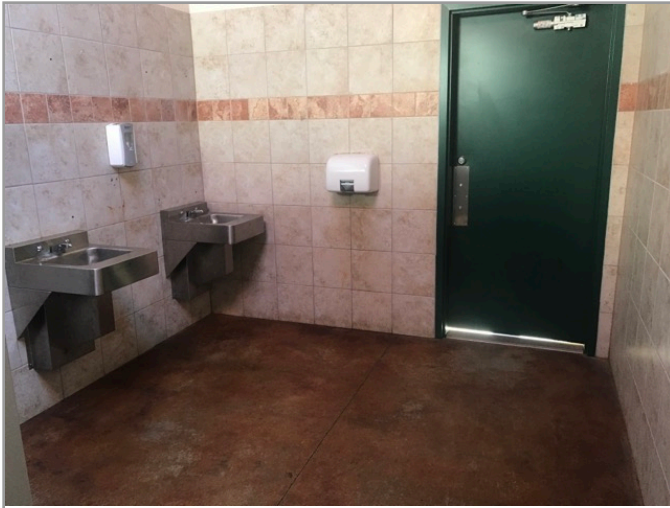
Toilet stall overview
