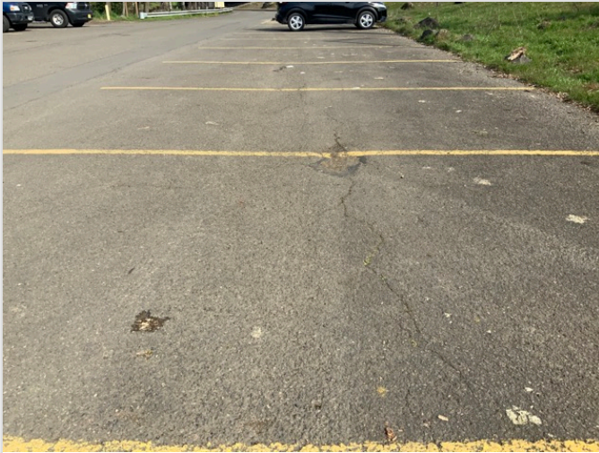
Overview of accessible parking area
