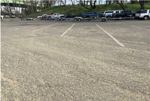
7 LOWER PARKING LOT, PAVEMENT, ASPHALT
