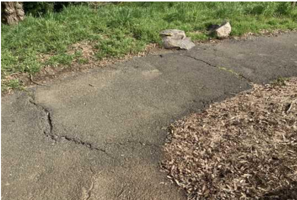
9 TRAIL SURFACE, ASPHALT, OVERLAY
