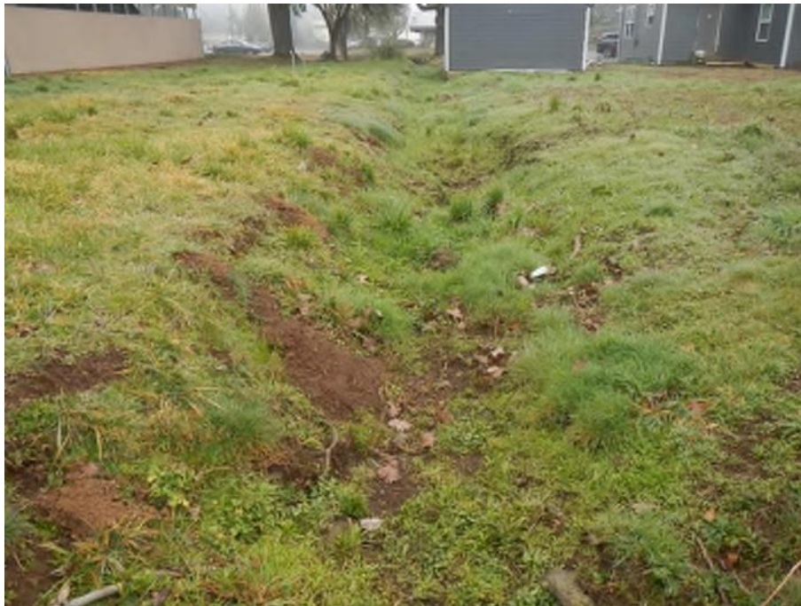
Photo 4. View looking south towards Warner Milne Road showing the channel of Drainage A next to the garage.
