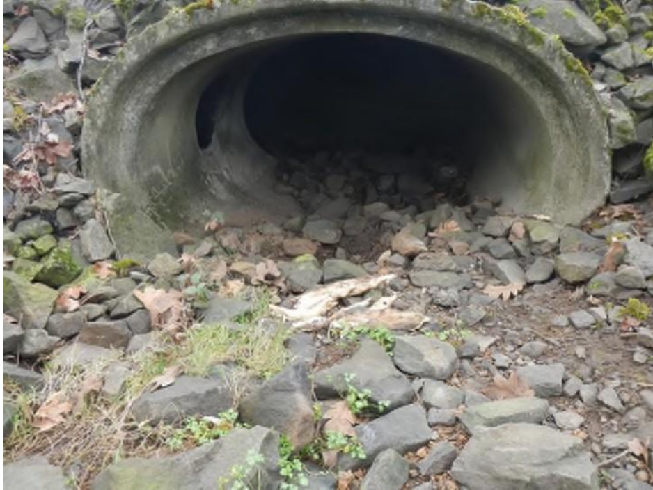
Photo 7. View looking south showing the inlet of the Warner Milne Road culvert.
