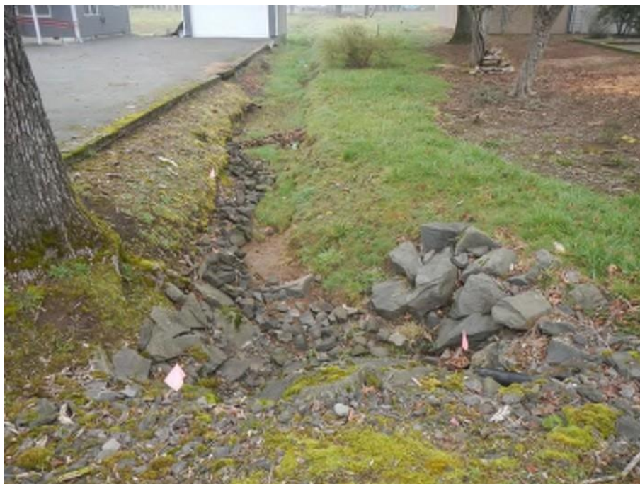
Photo 6. View looking north along Drainage A from the Warner Milne Road culvert.
