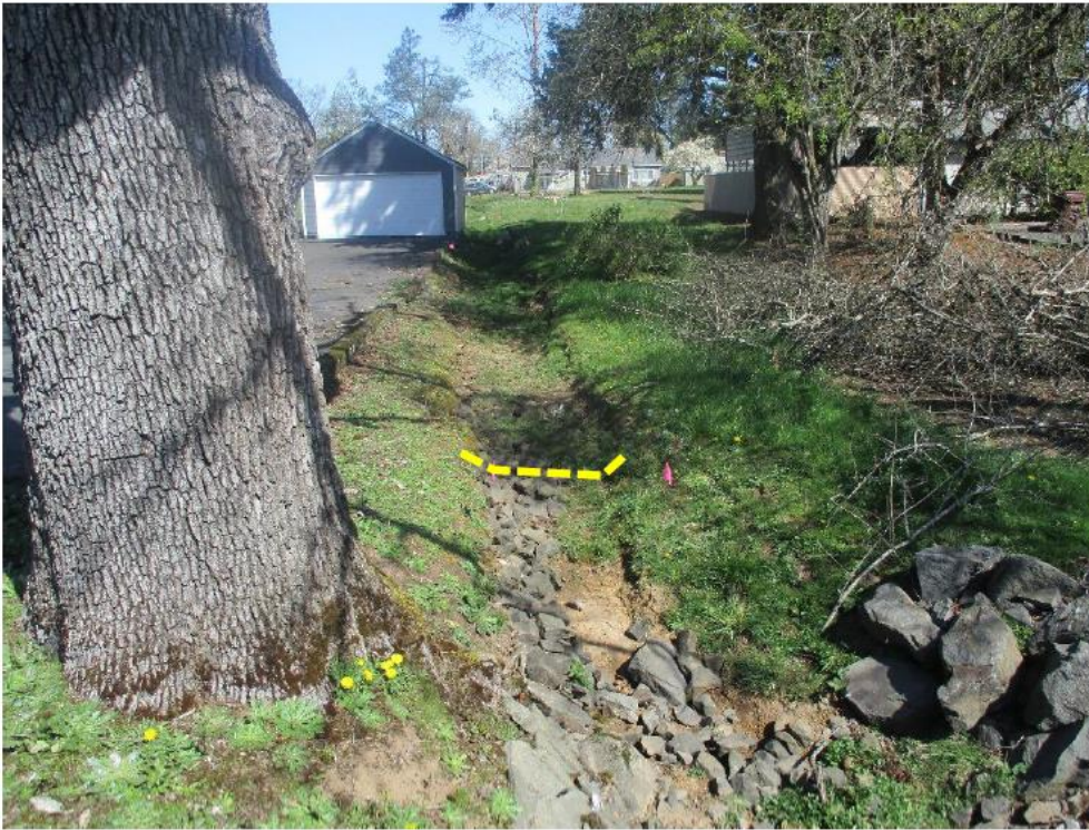
Photograph 10: View looking north, along Drainage A from the Warner Milne Road culvert. The downstream reach, with bare bed and riprap, can be seen in the foreground. The yellow dashes indicate the reach boundary. Photograph taken April 12, 2021.
