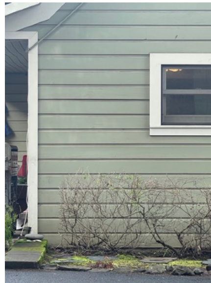
502 4th Ave Siding
