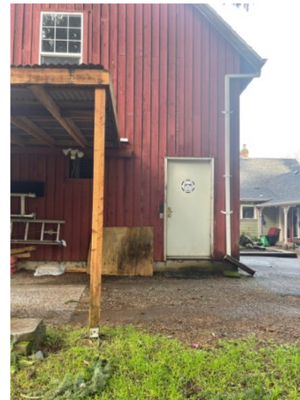
502 4th Ave Siding
