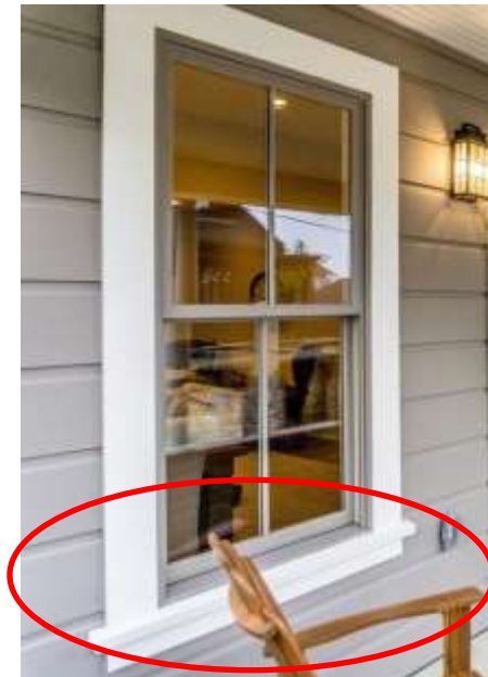
Figure 3. Window with "Stool" and "Apron"
