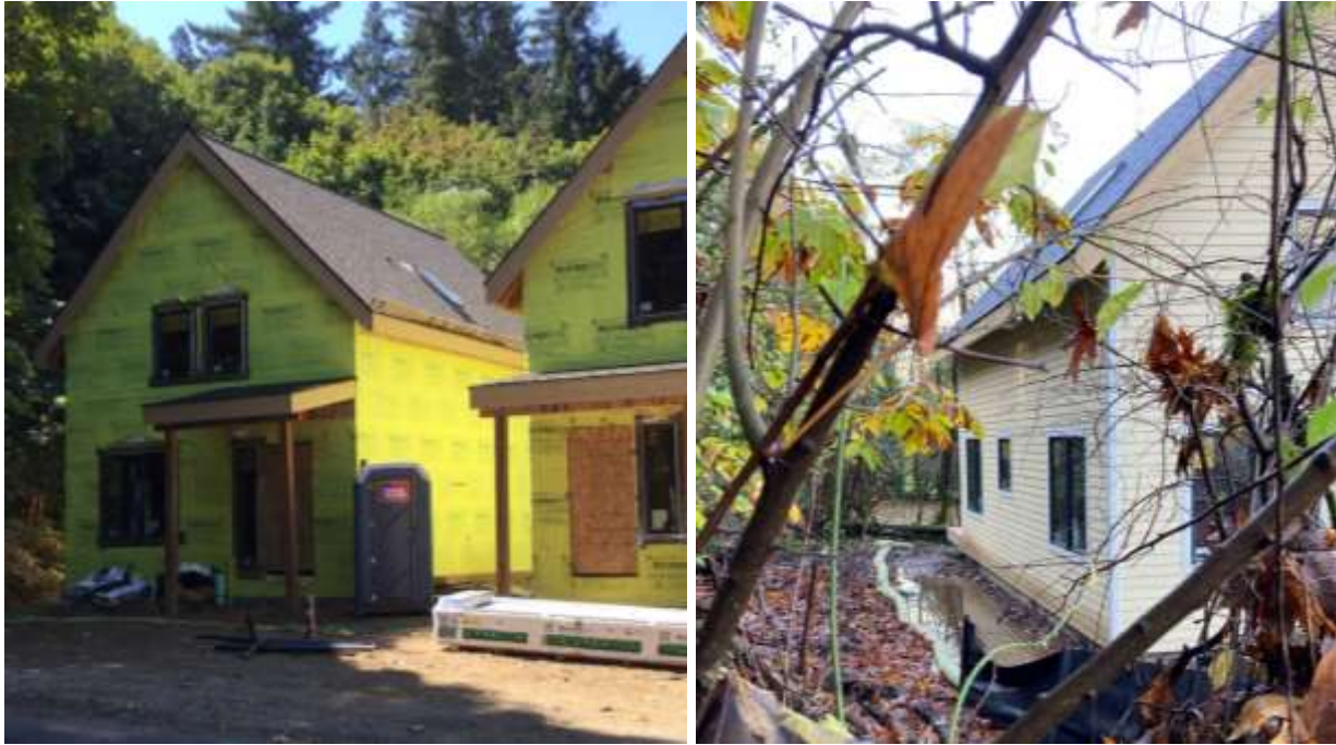
Figure 6. House #5 Skylight on north side (left) and south side (right)
