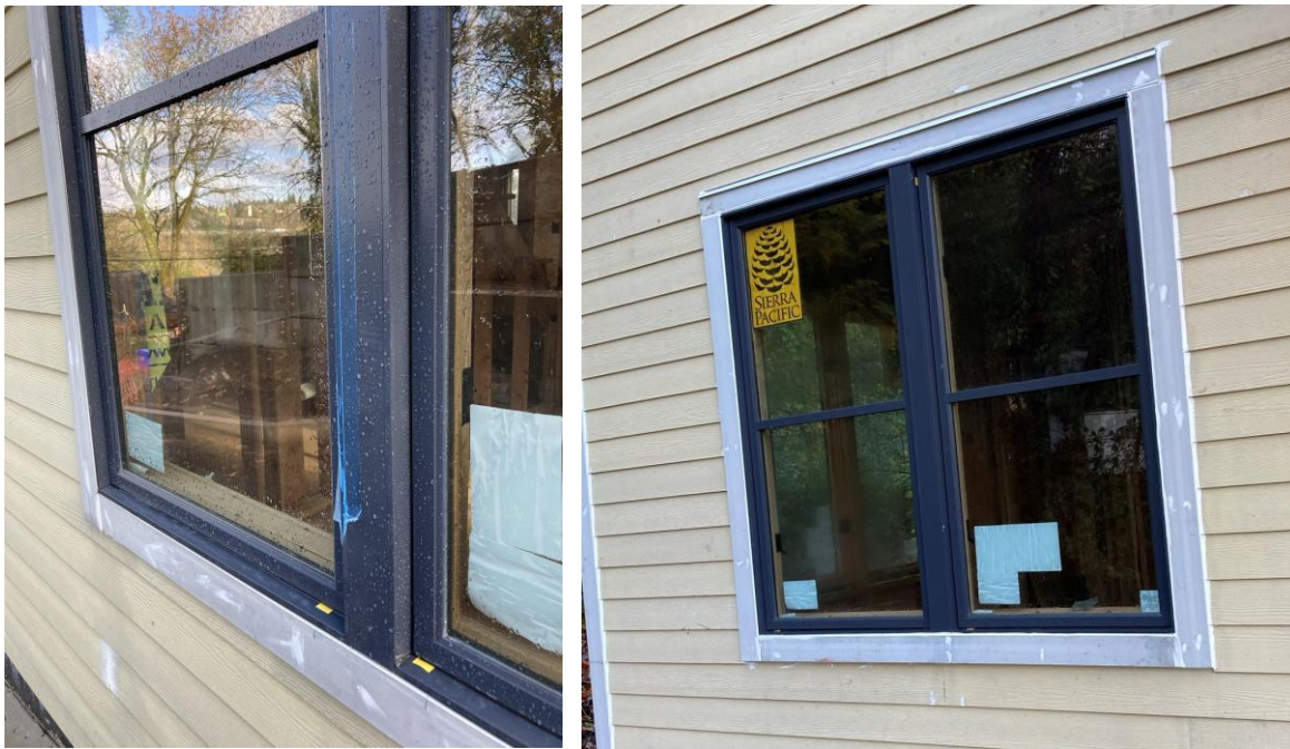
Figures 8 and 9. Casement windows with simulated divided lite.
