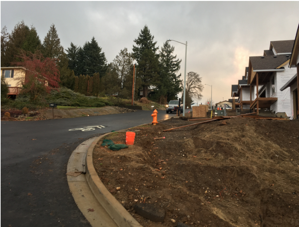
View from Laurel Ridge Avenue looking east along Cleveland Street
