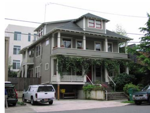
2 ½ Story Four Square Multifamily
