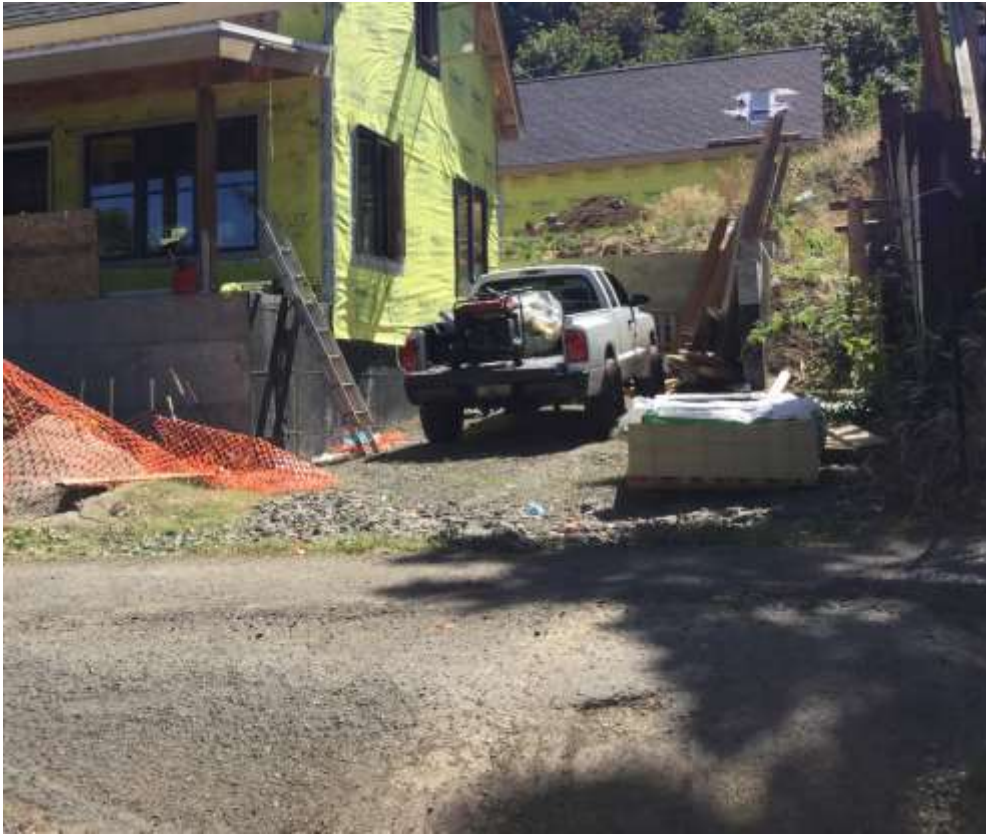
Retaining wall next to House #1, at end of driveway
