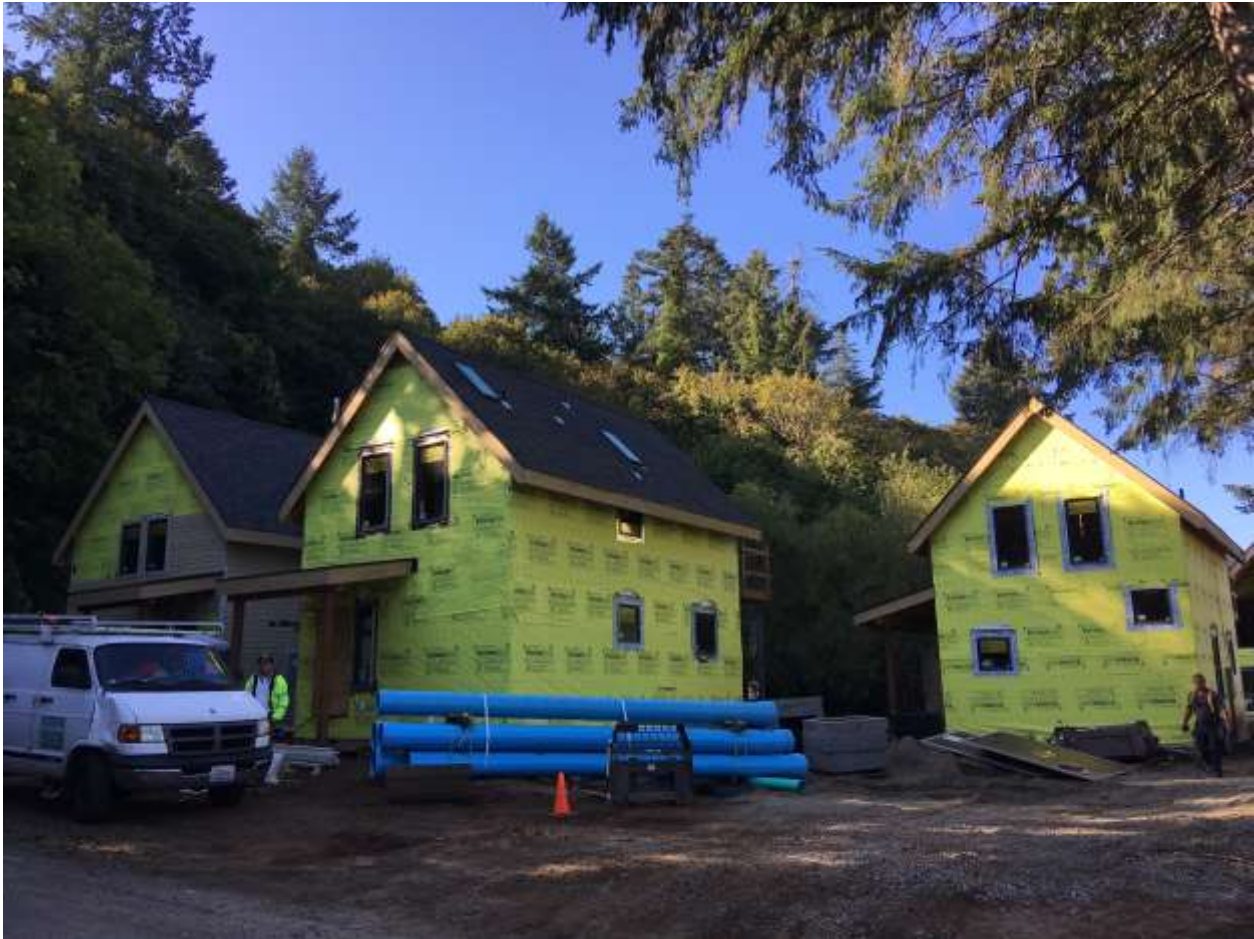
View from right-of- way on Miller Street – House #4 skylights are visible. August 2020
