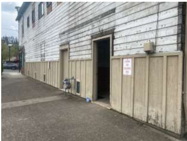
Figures 5 and 6. Front and side façades after asbestos siding removed by applicant
