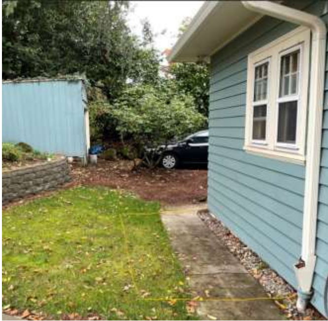
Existing condition on rear facade
