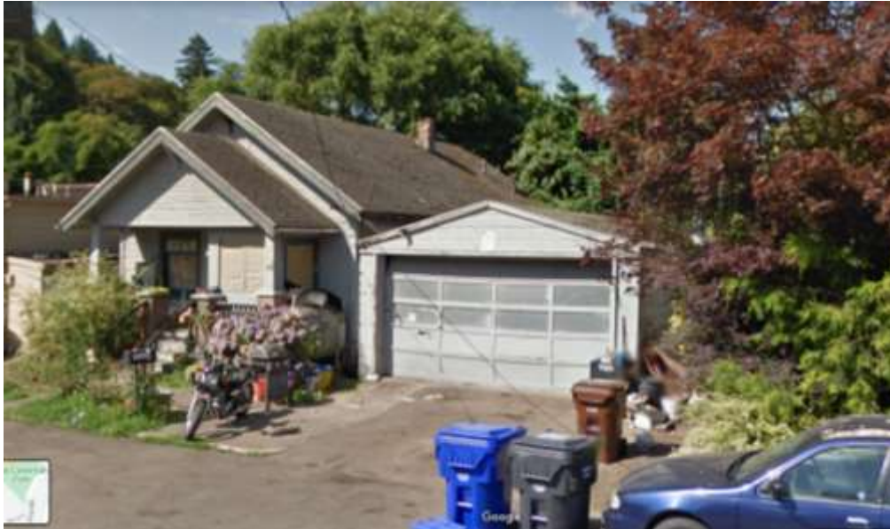
North roof plane where dormer is proposed.
