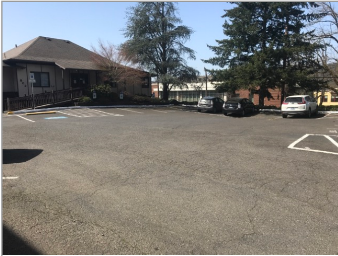
Overview of accessible parking area
