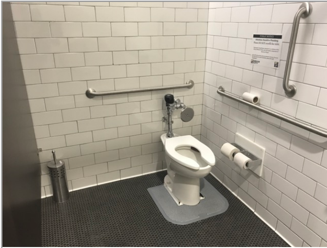
Toilet stall overview
