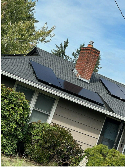
Panels installed on Beverly Dr.
