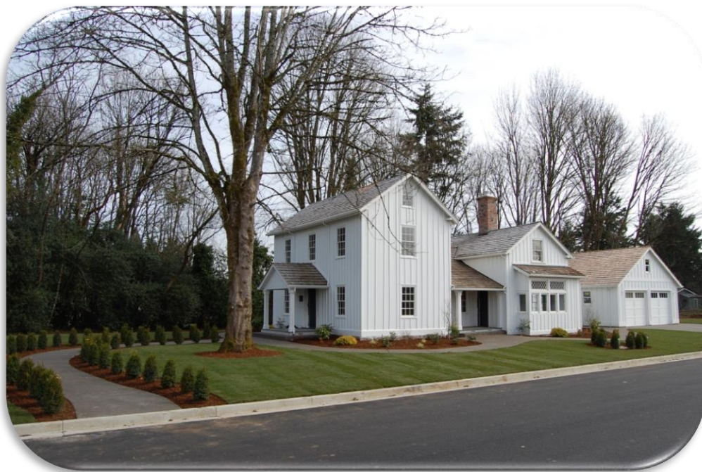
McCarver House 2008- New garage and kitchen addition
