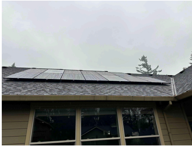
Panels installed on Charman St.
