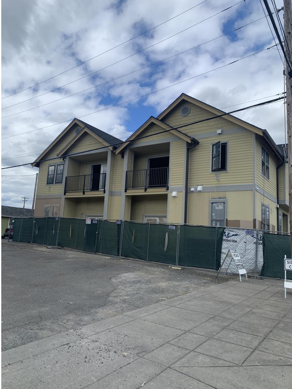
May 2024- Rear of Building from Monroe Street
