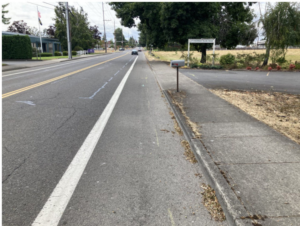
Warner-Milne Road looking west along the project frontage
