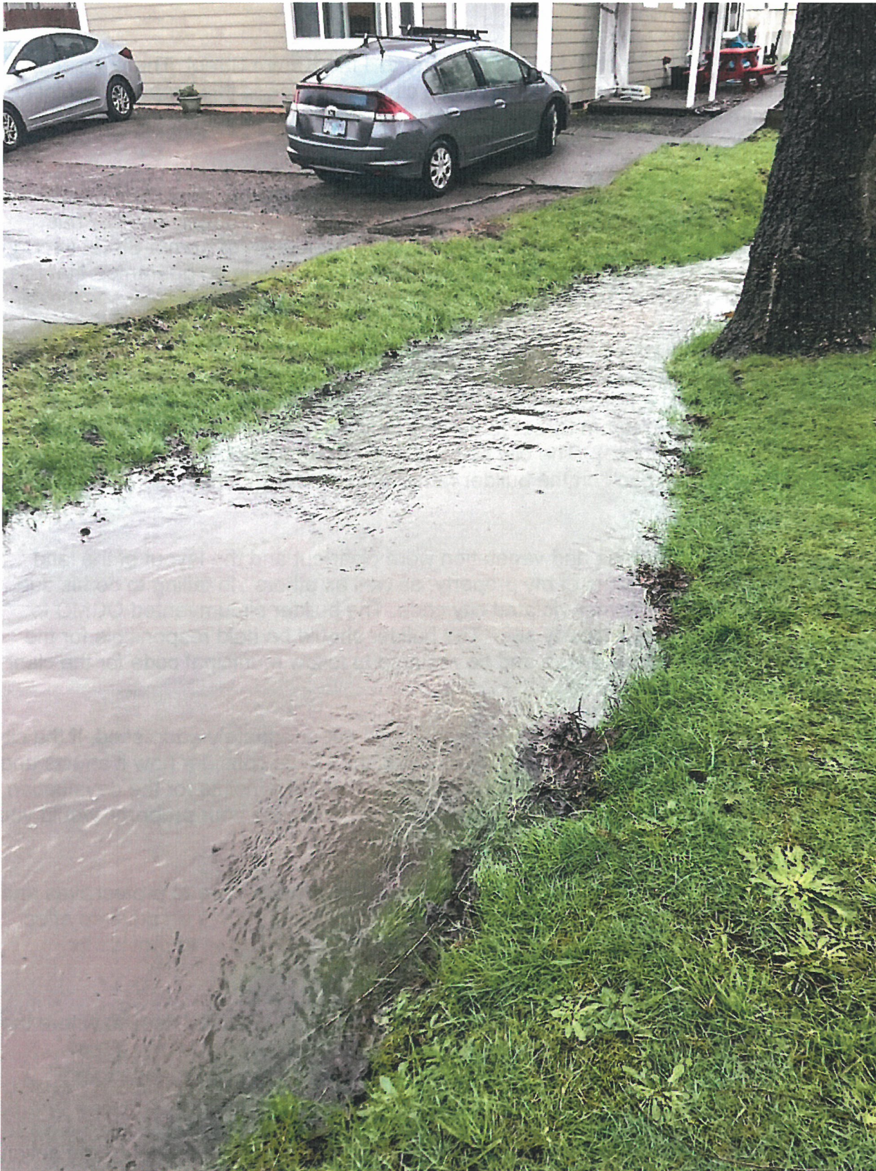
Image: Ditch near capacity at 1147 Kamm Street (January 2022).
