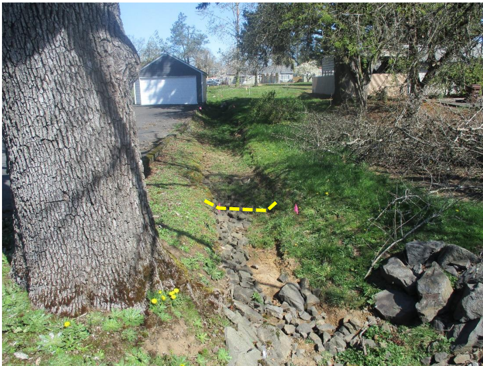
Photograph 10: View looking north, along Drainage A from the Warner Milne Road culvert. The downstream reach, with bare bed and riprap, can be seen in the foreground. The yellow dashes indicate the reach boundary. Photograph taken April 12, 2021.
