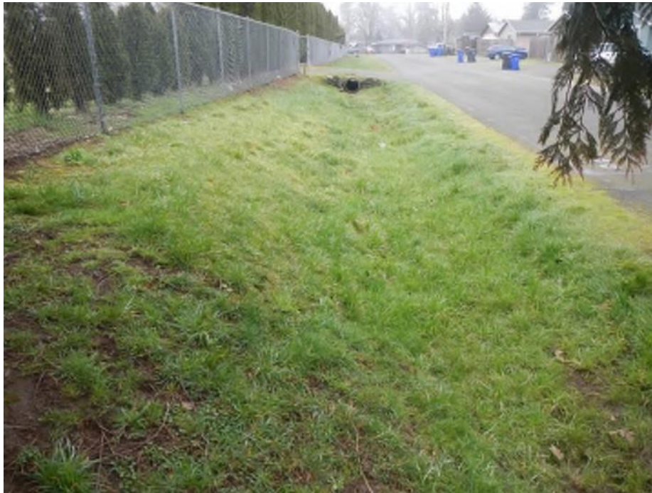
Photo 1. View looking north from end of the study area along Drainage A. Kamm Street is on the right.
