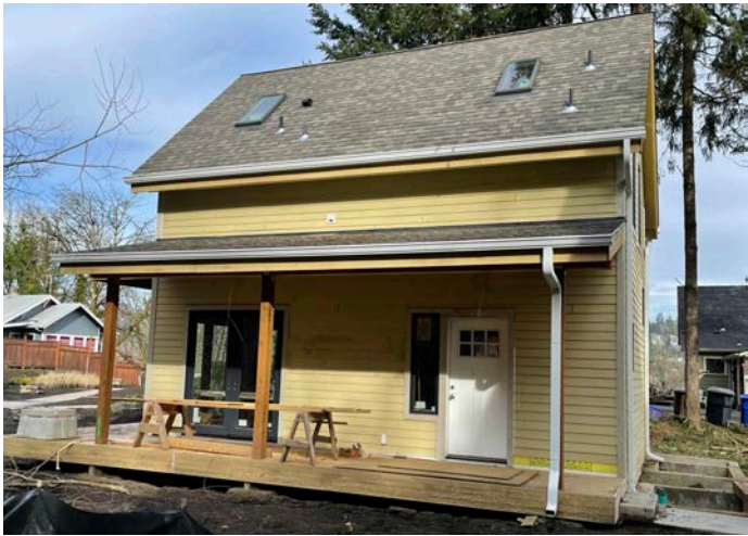
Permitted / As Built
