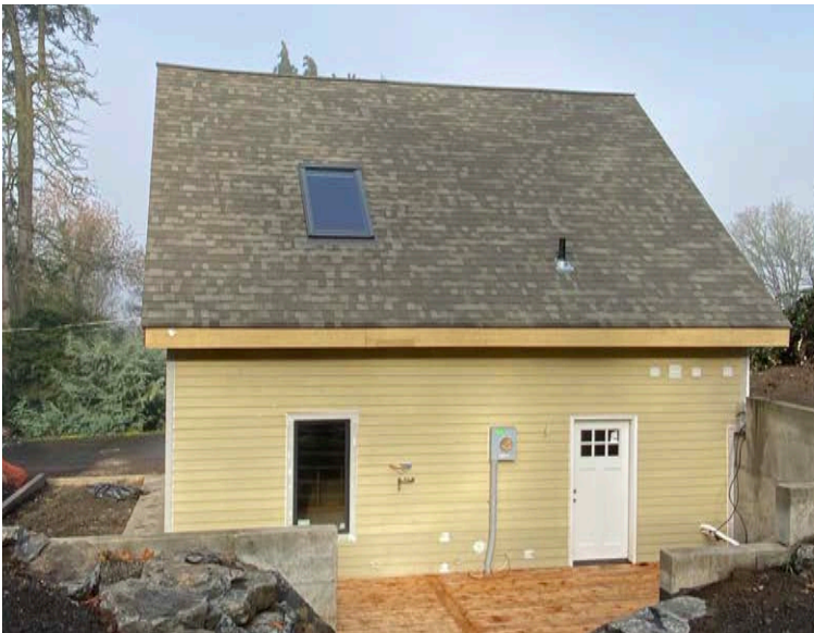
Permitted / As Built
