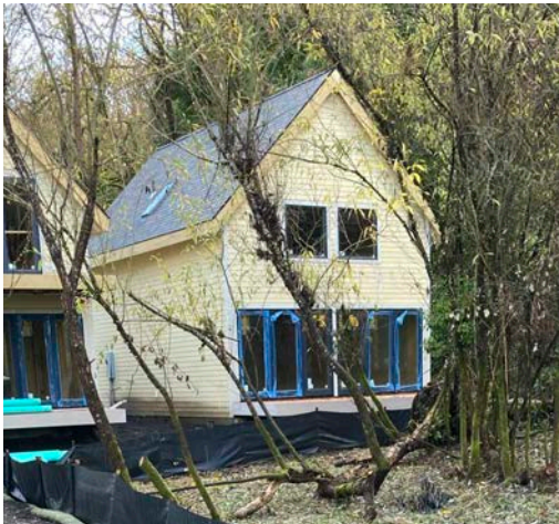
Permitted / As Built
