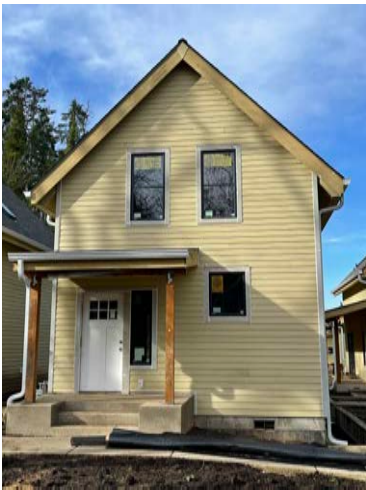
Permitted / As Built
