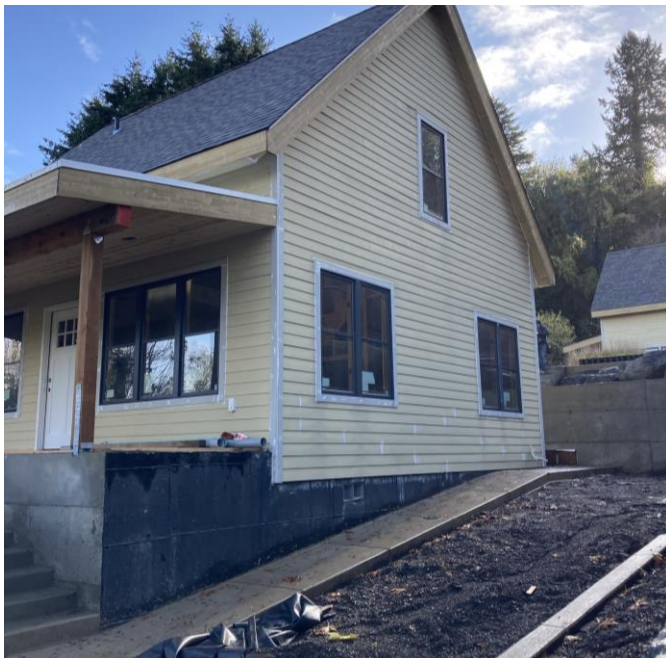
Figure 6. House #1 with retaining wall shown behind.
