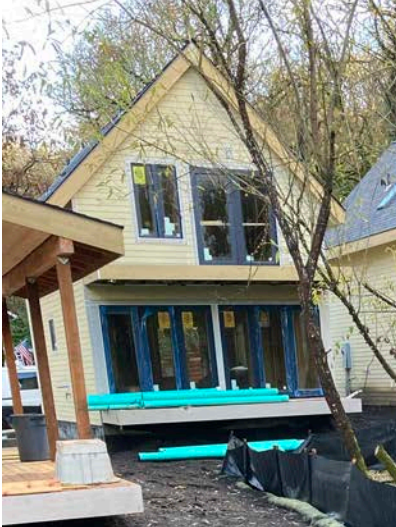
Permitted / As Built
