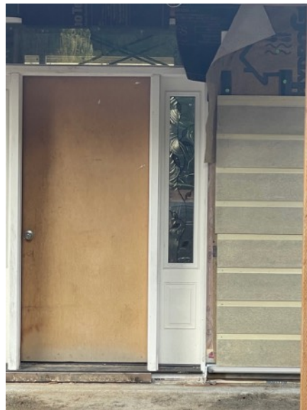
4th Ave New Home
