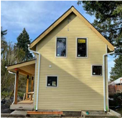
Permitted / As Built
