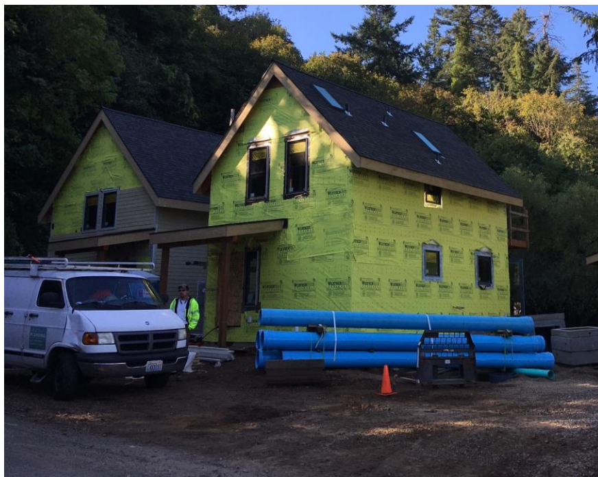
Figure 7. View from right-of-way on Miller Street – House #4 skylights are visible. August 2020
