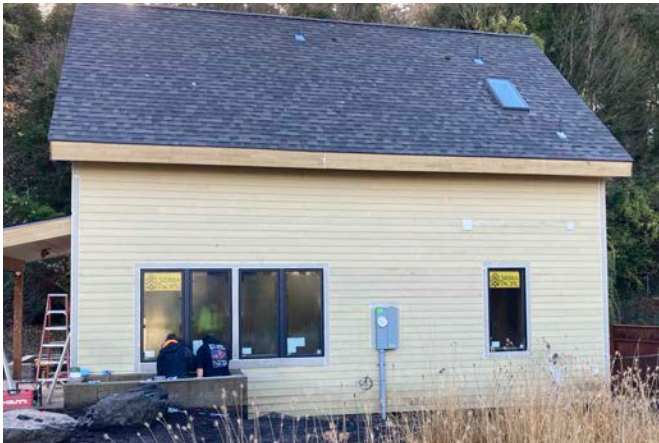
Permitted / As Built
