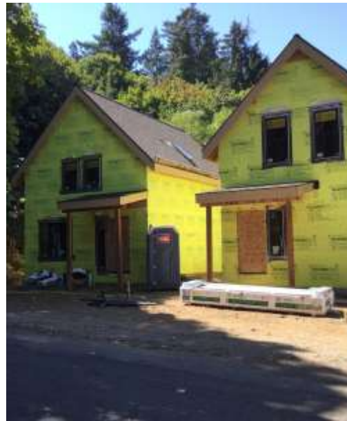
(Right) View from right-of- way on Miller Street – House #5 skylight. August 2020
