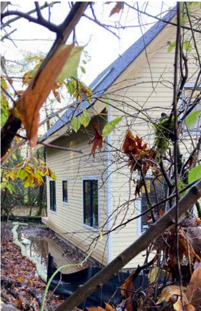
Permitted / As Built
