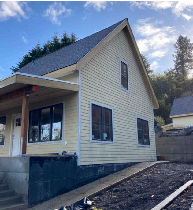
Permitted / As Built
