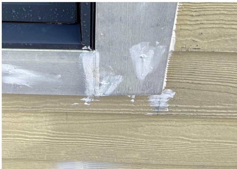
Figure 3. Textured fiber cement (hardieboard) siding on the constructed House #1.
