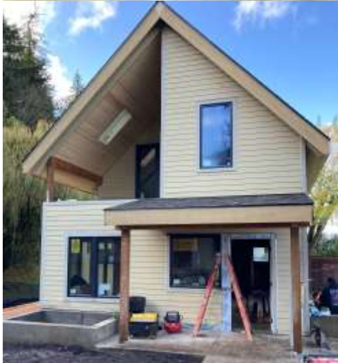
Textured fiber cement (hardieboard) siding on the constructed homes.
