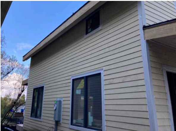
Permitted / As Built
