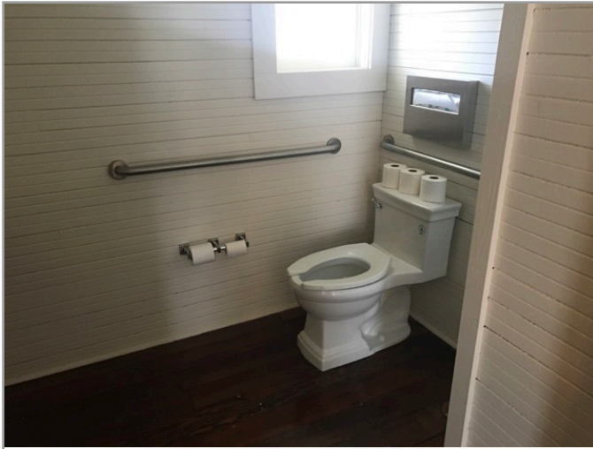
Toilet stall overview
