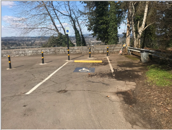
Overview of accessible parking area
