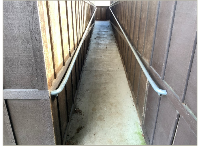
2 – RAMP TO BUILDING ENTRANCE
