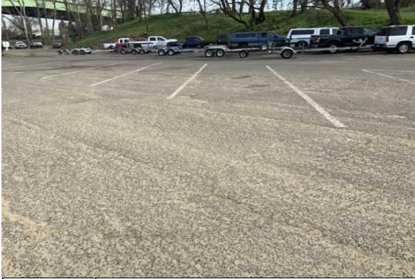
7 LOWER PARKING LOT, PAVEMENT, ASPHALT
