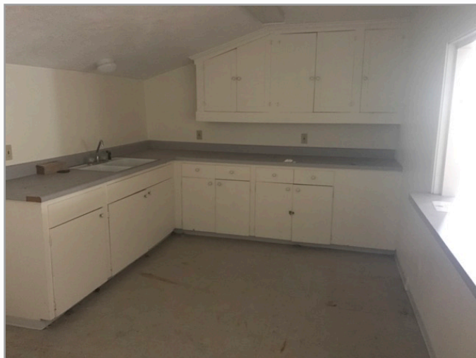
Kitchen cabinets/sink clearance
