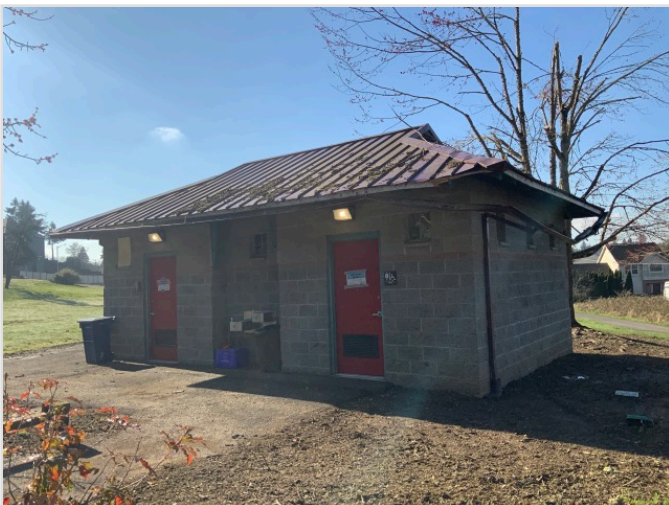
Toilet stall overview
