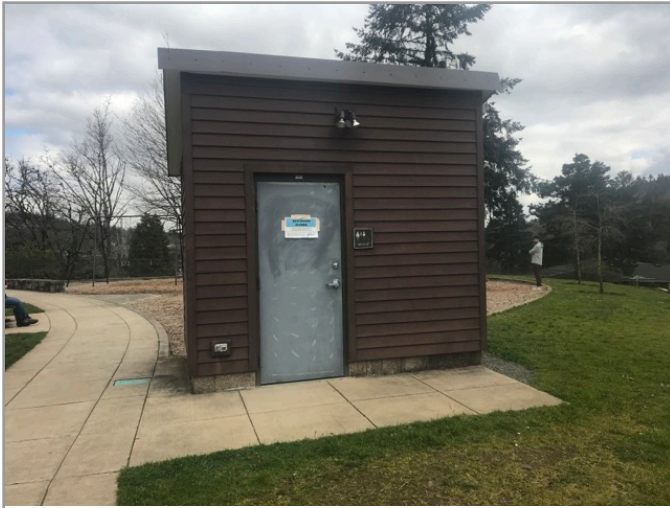
Toilet stall overview
