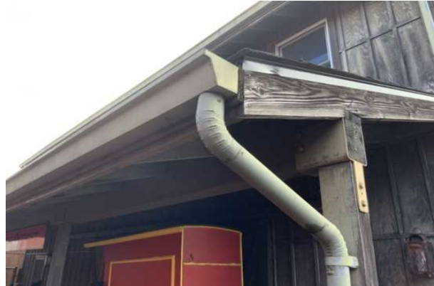
14 GUTTERS AND DOWNSPOUTS
