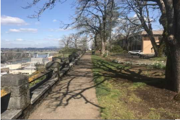
1 OVERVIEW OF THE SIDEWALK
