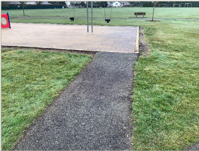
9 - ACCESSIBLE ROUTE TO PLAYGROUND
