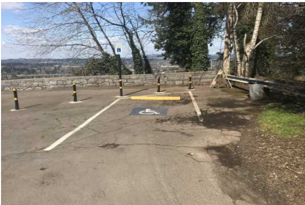
5 OVERVIEW OF ACCESSIBLE PARKING AREA
