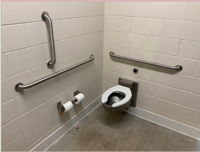
7 - ACCESSIBLE RESTROOM ACCOMMODATIONS
