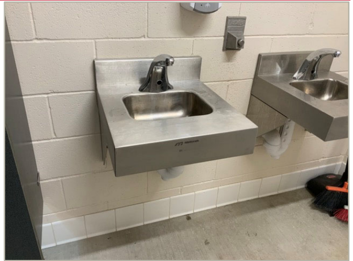
8 - ACCESSIBLE RESTROOM ACCOMMODATIONS
