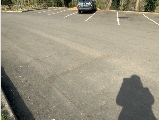
Overview of accessible parking area
