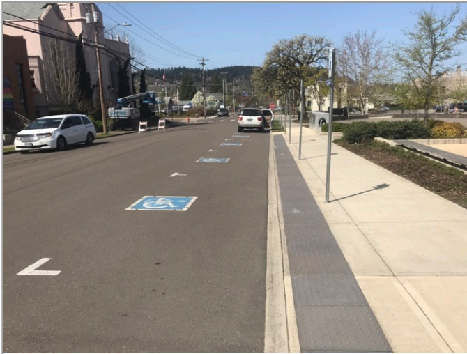
Overview of accessible parking area
