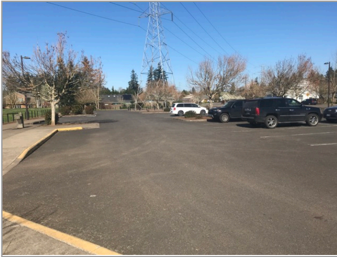
Overview of accessible parking area
