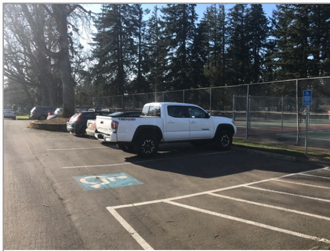
Overview of accessible parking area
