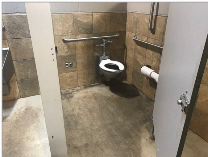
Toilet stall overview
