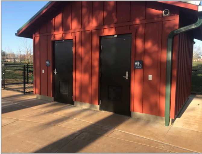
Toilet stall overview
