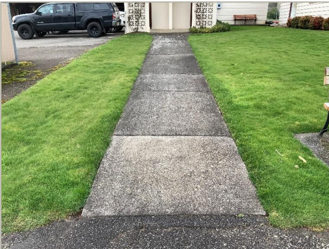
3 – EXTERIOR PATH OF TRAVEL TO BUILDING ENTRANCE
