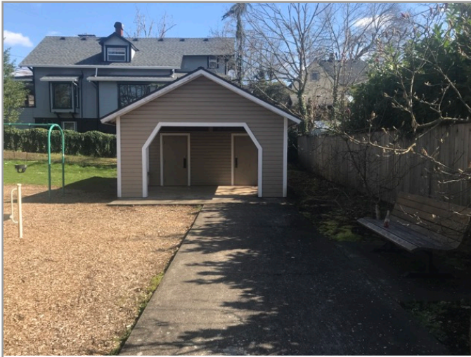
Toilet stall overview
