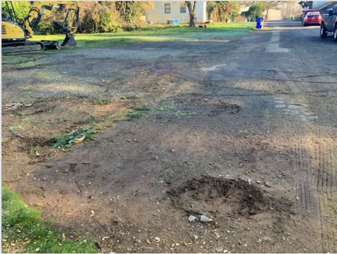
Overview of accessible parking area
