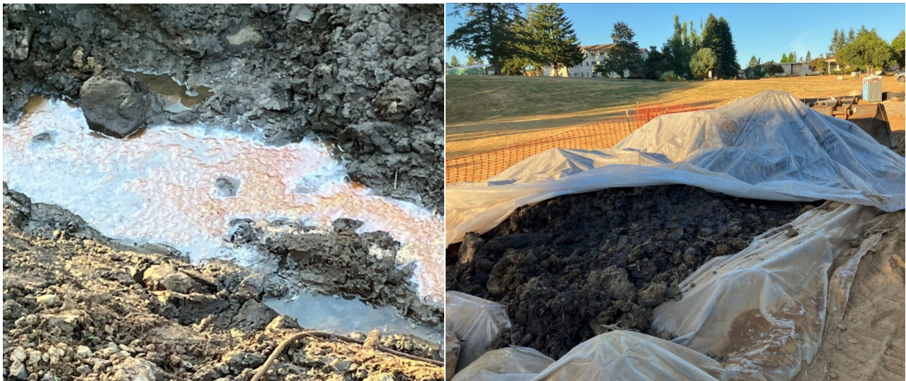
Figure 2 images of initial contamination (top) and excavated soil (bottom) discovered in August of 2022. DEQ was satisfied with the mitigation plan and approved the completion of construction.
