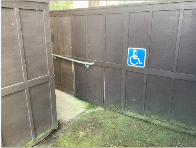
1 – EXTERIOR ACCESSIBLE PATH
