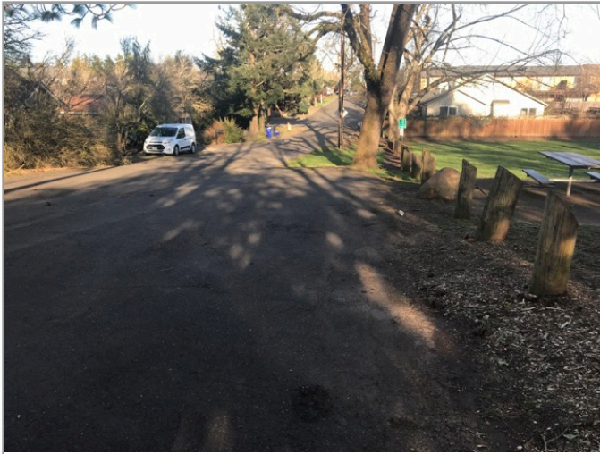
Overview of accessible parking area
