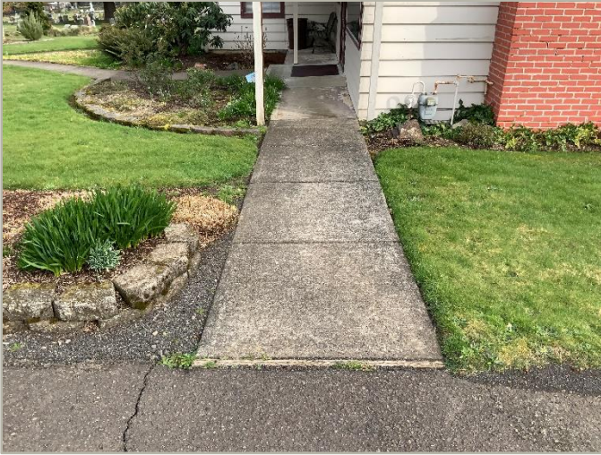
1 – EXTERIOR PATH OF TRAVEL TO BUILDING ENTRANCE
