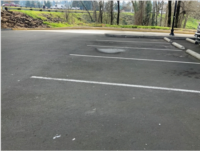
Overview of accessible parking area
