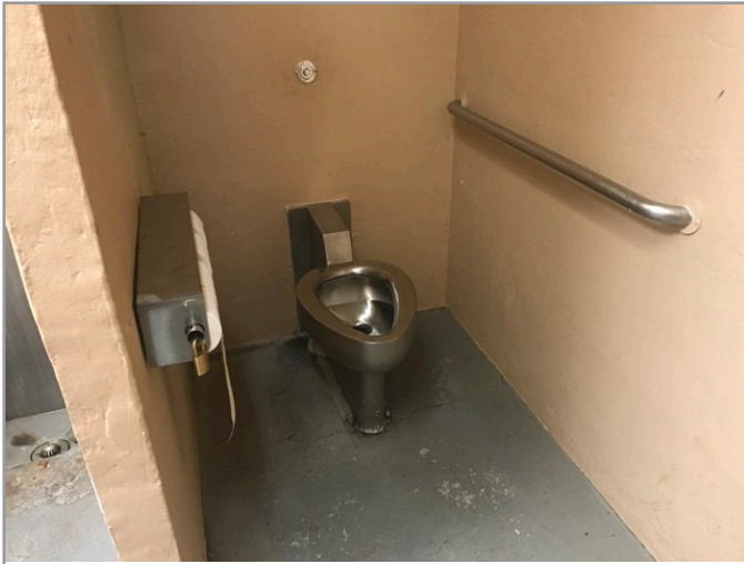
Toilet stall overview
