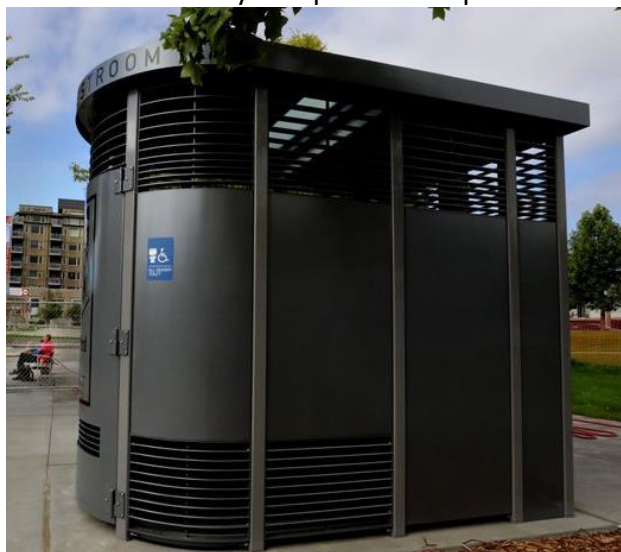
Portland Loo installation in Seattle, WA.
