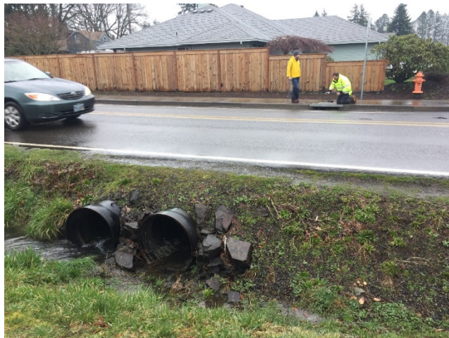
Figure 2: Inlet of culverts west of Leland Road
