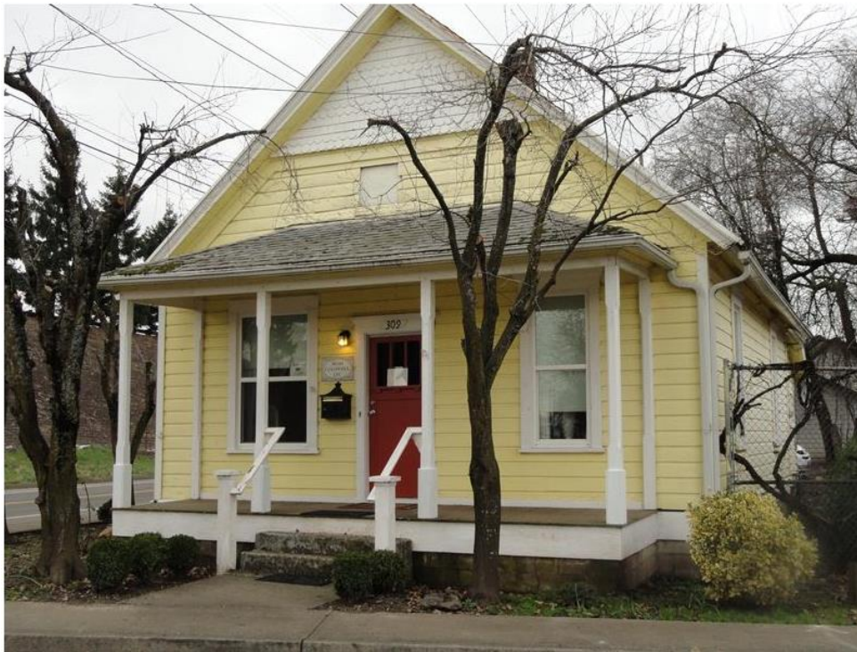
Figure 3. Front of structure during recent use as an office.
