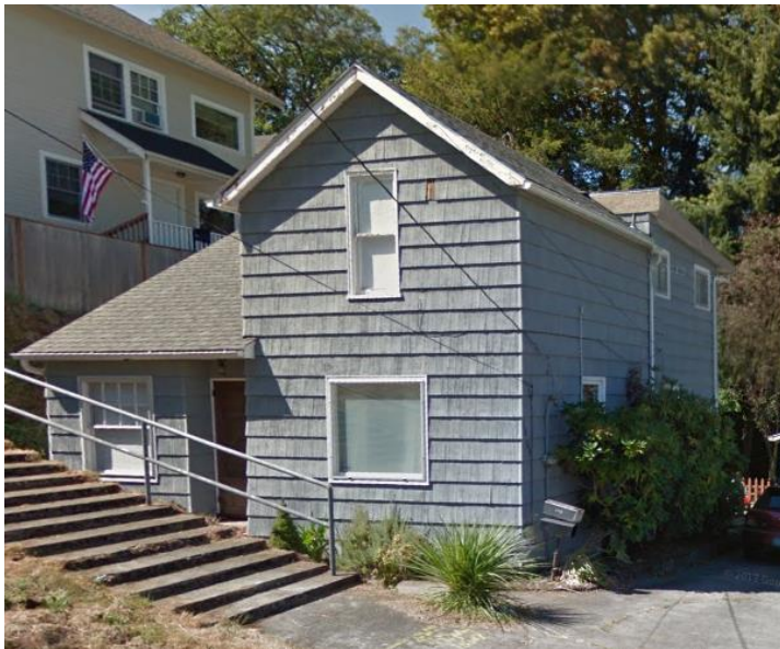
Existing house on site (non-designated).
