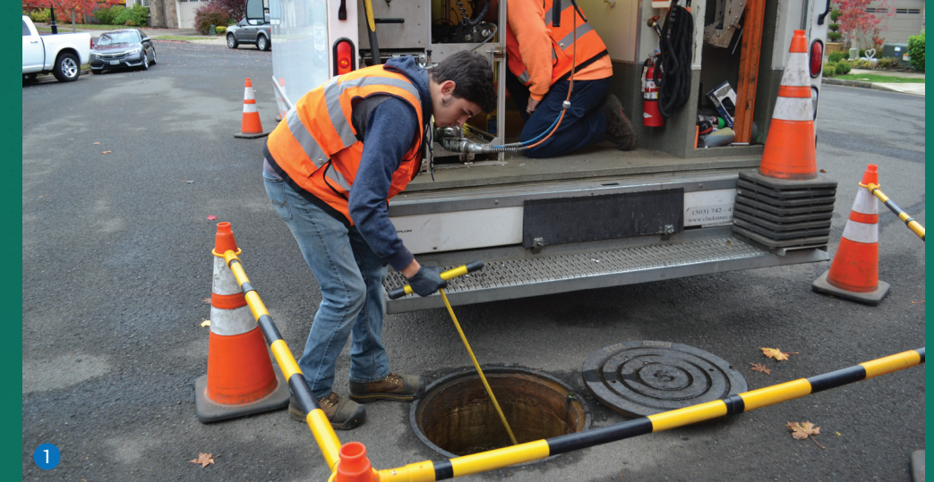
1 WES field operators inspect the pipes
