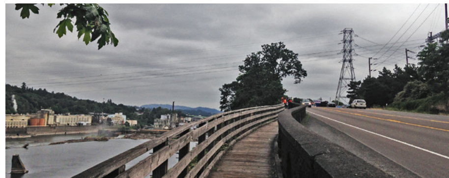
P-1 | McLoughlin Blvd boardwalk, looking north
