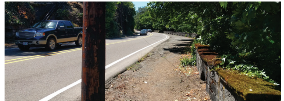
S. High Street, existing shoulder, looking south
