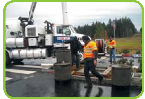
BayFilter System Cleanout
