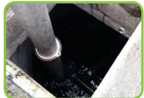
Jet Vactoring Through Access Hatch
