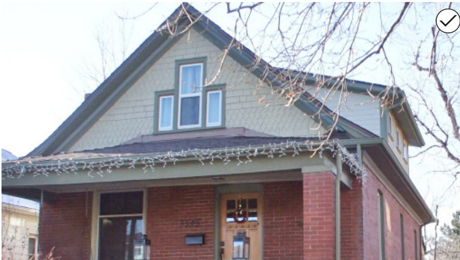
27. Design a dormer to be subordinate to the overall roof mass and in scale with those on similar historic structures. The dormer is set back behind the overhanging roof eave and the adjacent brick wall plane.
