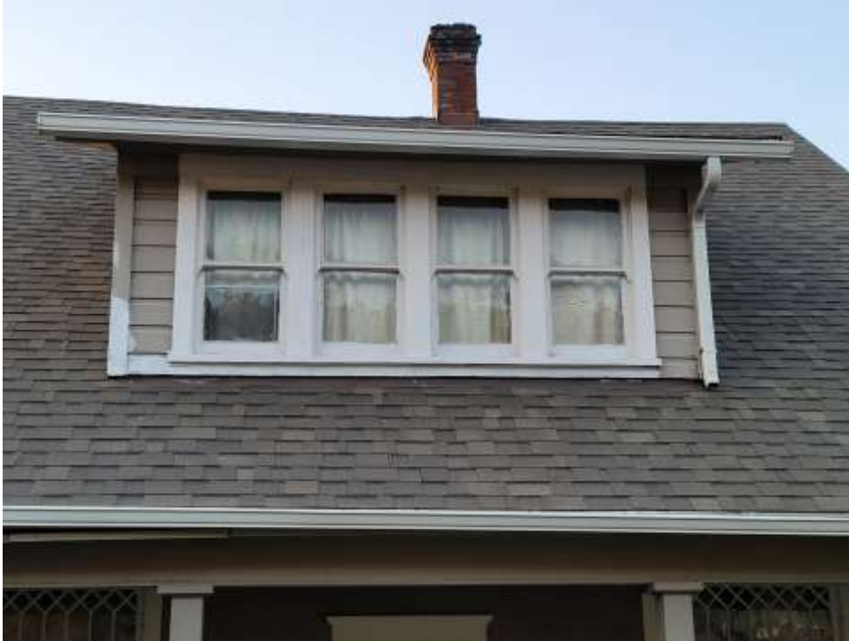
Photo of dormer on neighboring home. The owner wishes to replicate the look of the dormer on the North side of the home.
