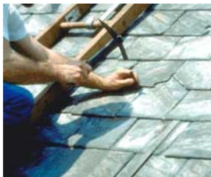
Repairing slate roof using traditional methods.
