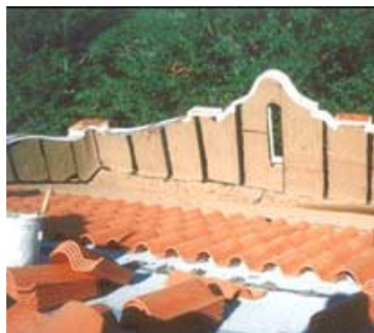
Replacement of damaged clay tile roof.
