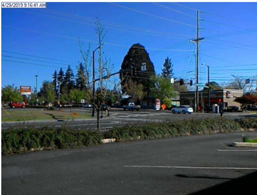
Site Overview from South facing Northeast
