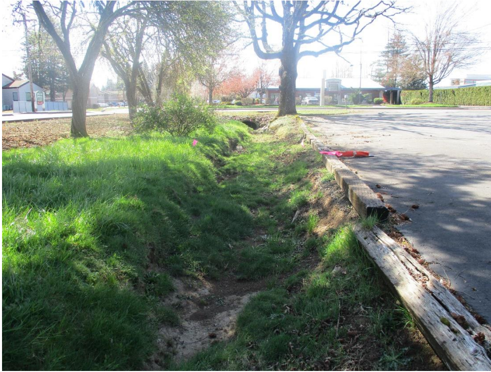
Photograph 9: View looking south towards Warner Milne Road showing the lower end of the upstream reach. A bare patch in the channel, scoured out by parking lot runoff following storm events can be seen in the foreground. Photograph taken April 12, 2021.
