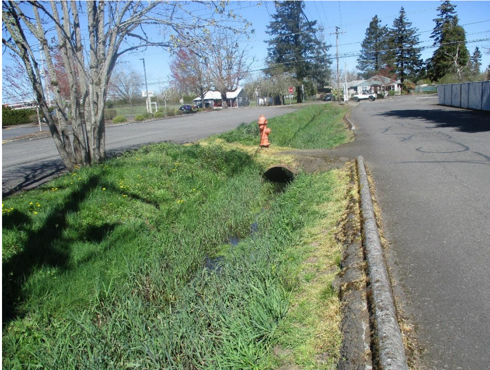
Photograph 13: View to the north towards Warner Milne Road showing Drainage A south of the study area. Standing water can be seen in the channel. Photograph taken April 12, 2021.
