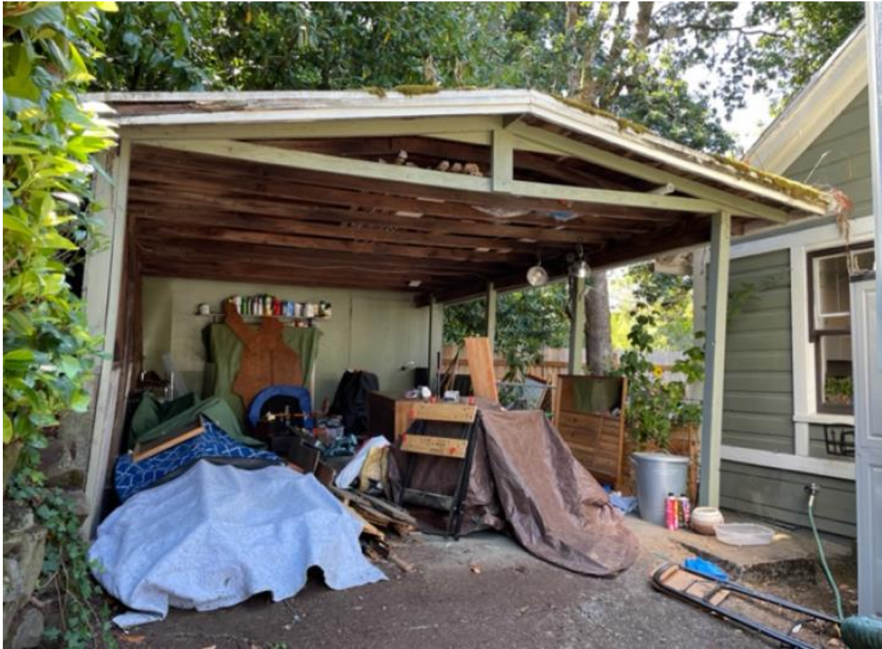
Close up view of carport
