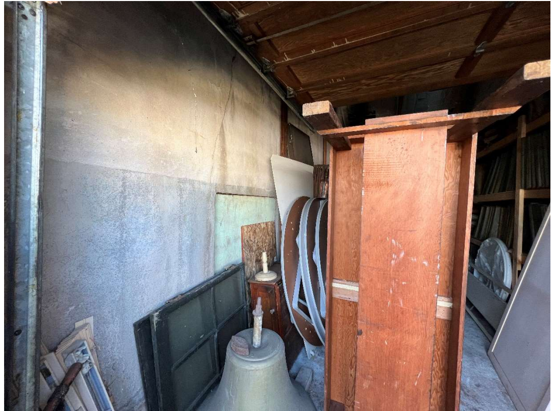
Interior of Garage addition, showing exterior wall of The Hive Social (no independent wall at the north side)
