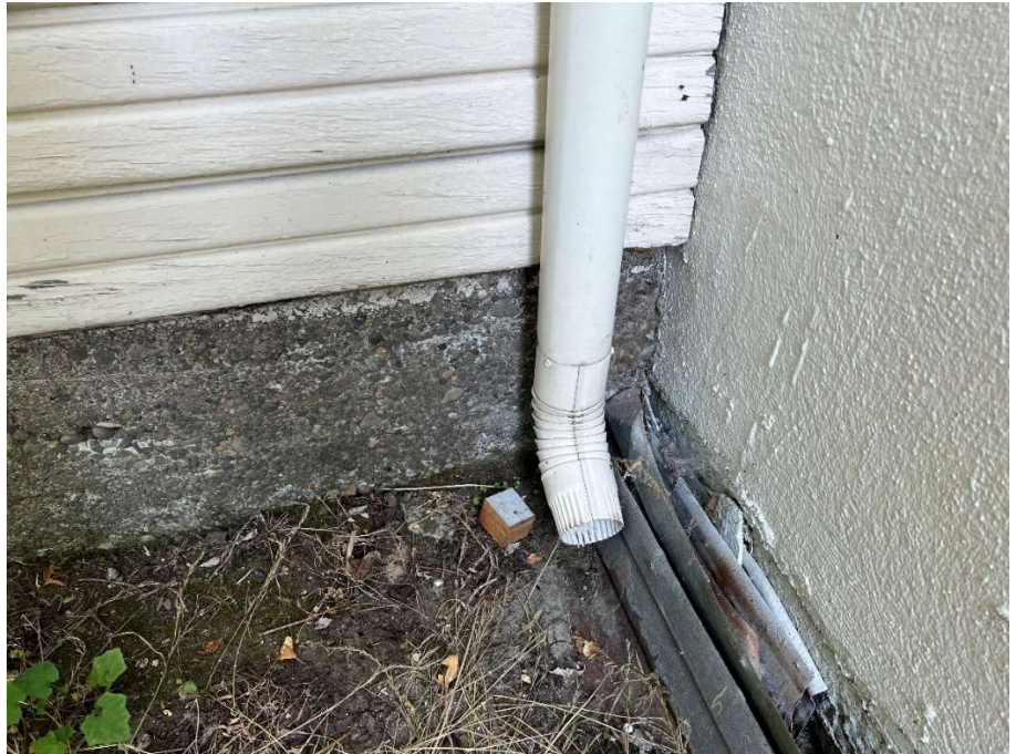
Downspout location adjacent to The Hive Social building wall
