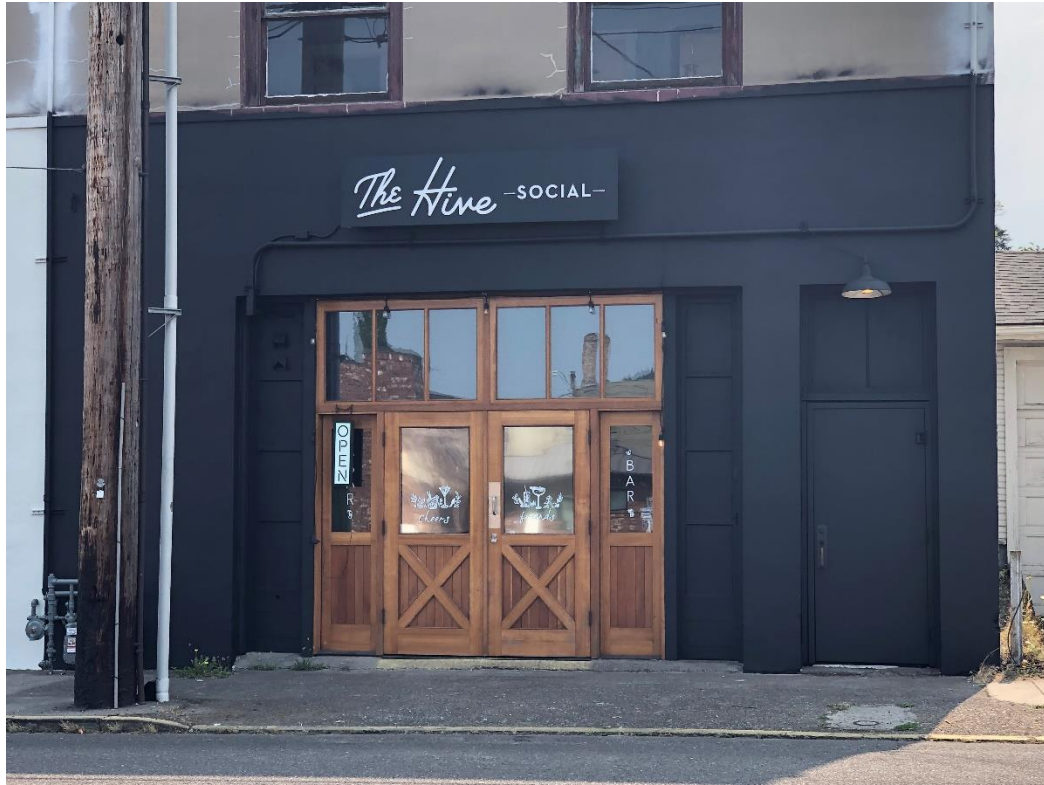
Washington Street view from the NW
