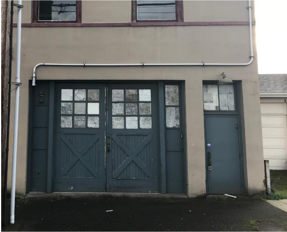
Conditions in 2019, prior to door replacement
