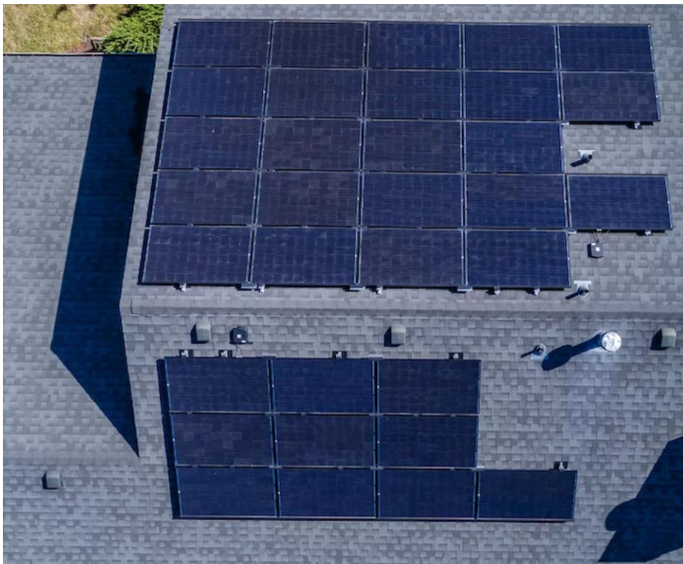
Image of Blue Raven solar installation (from Blue Raven website)
